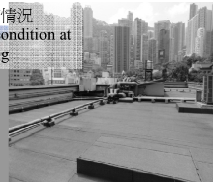
東座現有情況 Existing condition at East Wing
