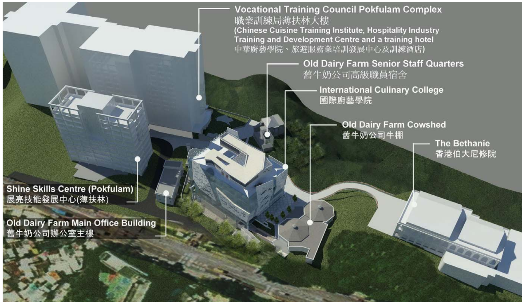
Aerial View of International Culinary College and Surrounding Buildings (2)
