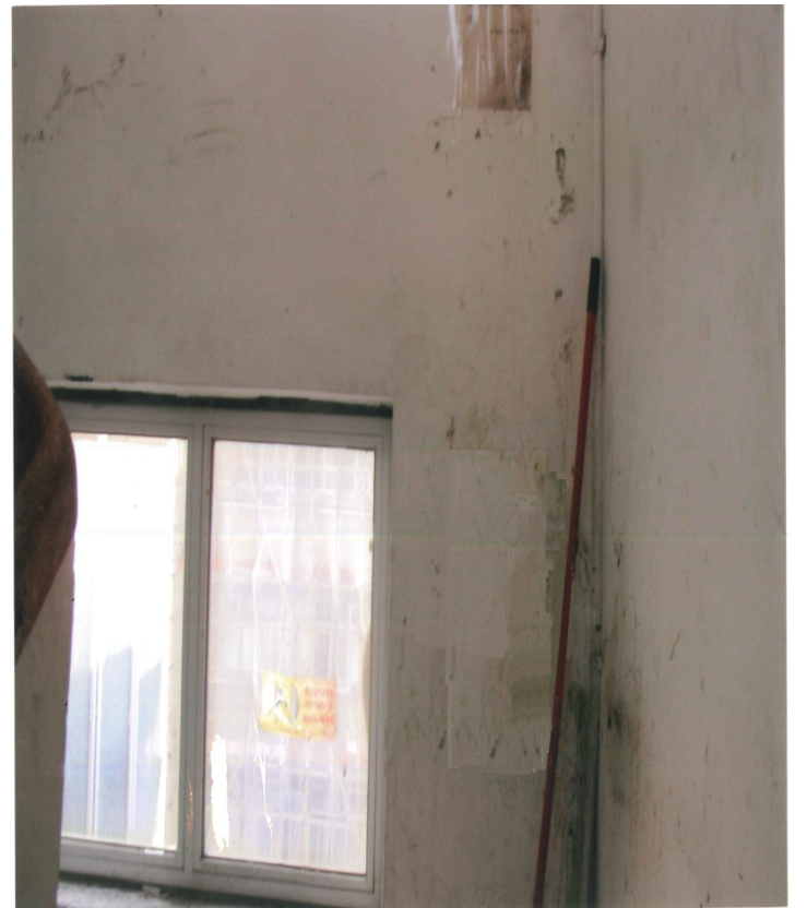
Staircases and fire escape – 5 th floor (after clearance)
