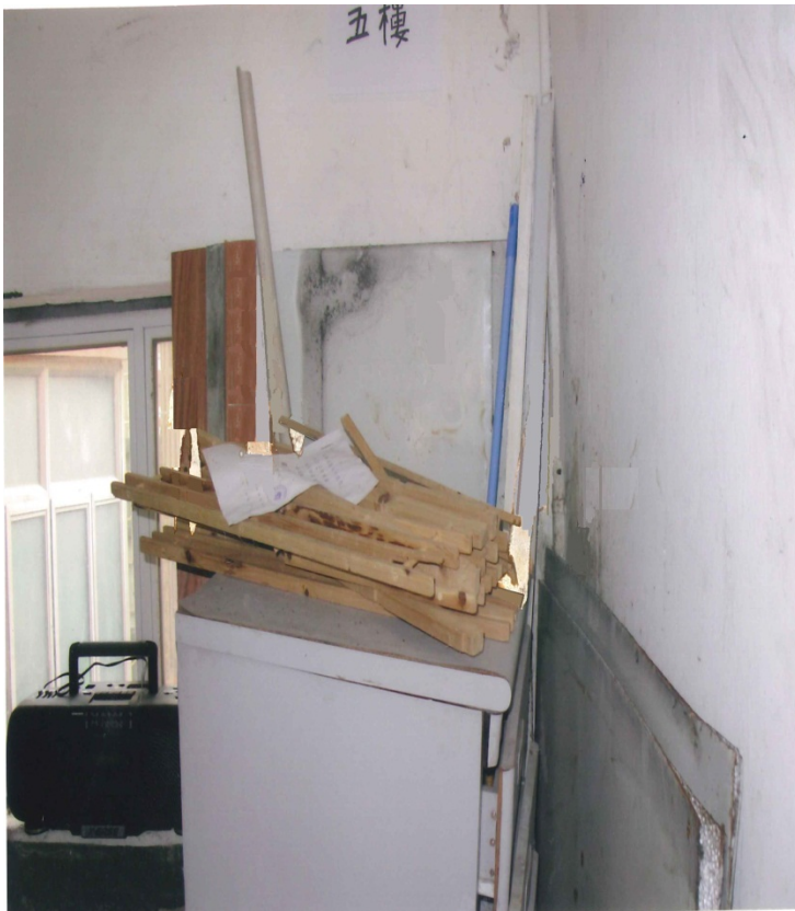
Staircases and fire escape – 5 th floor (before clearance)
