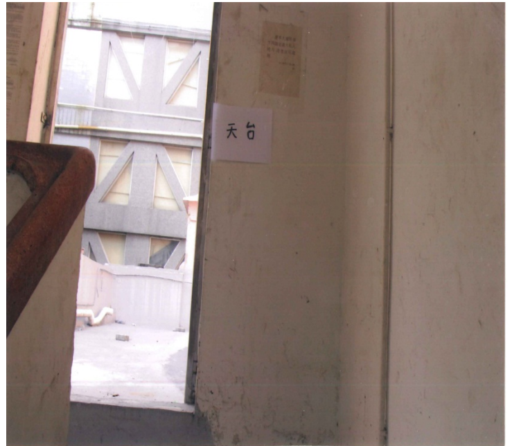
Staircases and fire escape – the roof (after clearance)
