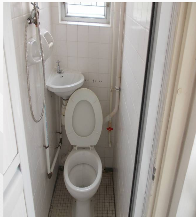
After modification works
