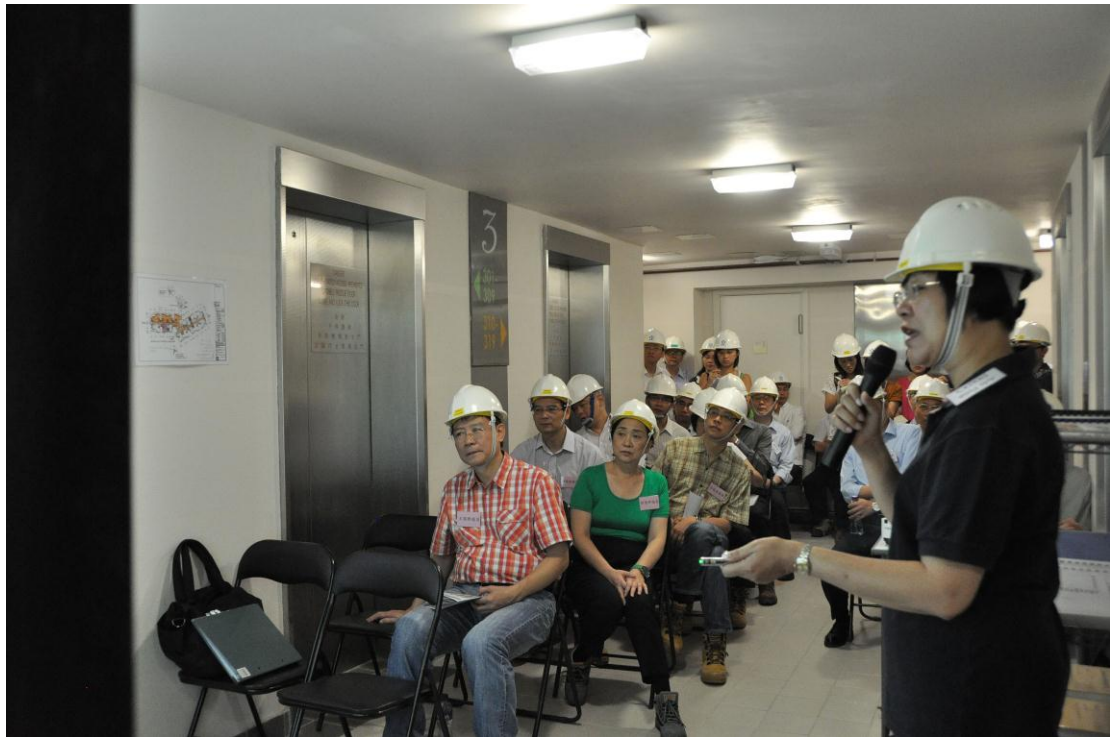
LegCo Members receive a briefing on site safety and quality management from Ms Ada FUNG (right), Deputy Director (Development & Construction) of Housing Department, at the construction site of Public Rental Housing Development at Tseung Kwan O Area 65B.
