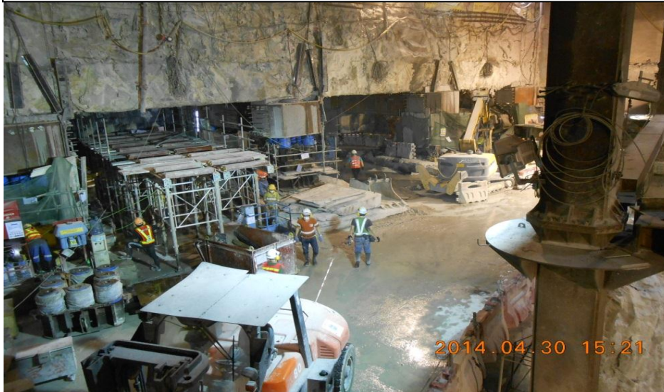
港島綫隧道支撐架橫樑安裝 Island Line underpinning beam installation
