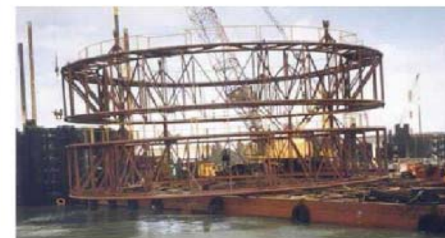
D. TEMPLATE USED TO STABILIZE CIRCULAR CELL
