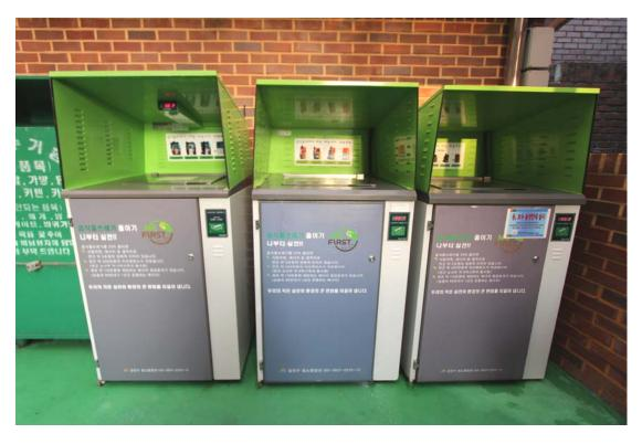
Collection bins installed with RFID chips to keep track of food waste generation by individual households
