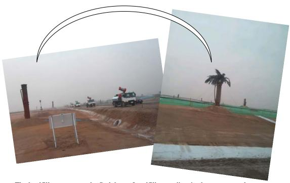
The landfill gas vents at the Sudokwon Landfill were disguised as trees; trucks were spraying pesticide onto the Landfill
