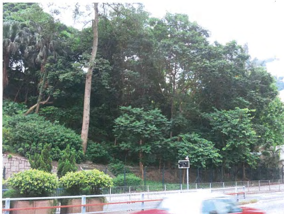
E.4 View from Cotton Tree Drive of slope on north- western side of Flagstaff House at the area where the pumping station is proposed.
