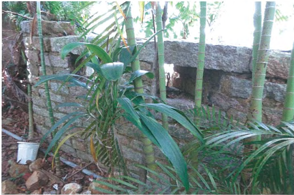
E.9 View from inside of the historic defensive wall of the group of two loopholes facing in a roughly westerly direction. These loopholes would enable enfilade fire to be brought on any attacking soldier approaching the section of wall running approximately west from the corner.
