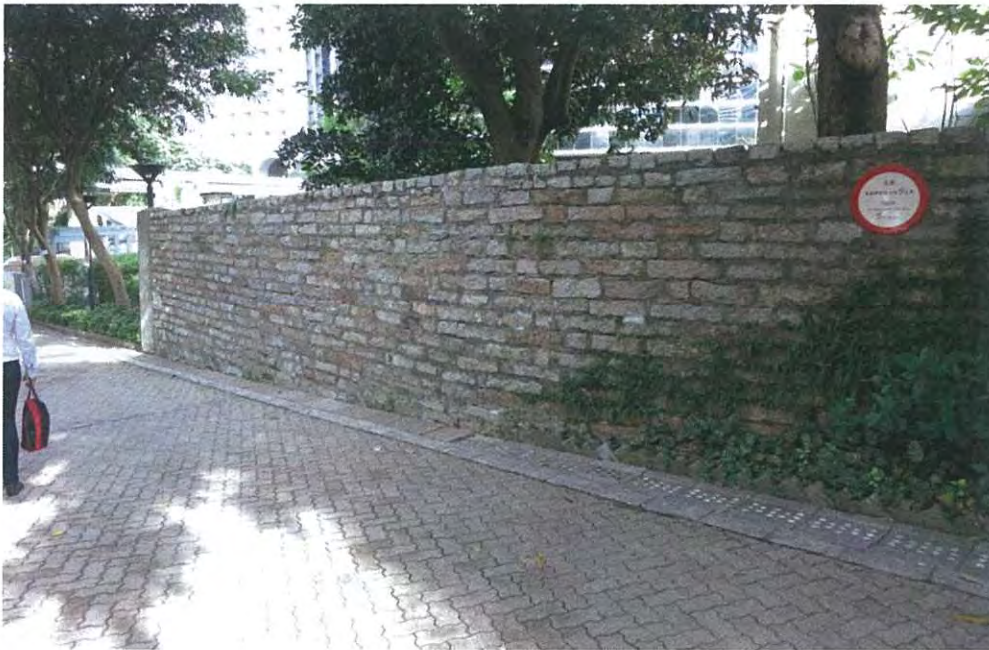
E.6 South-western end of historic defensive squared rubble masonry wall in Hong Kong Park to the south-west of Flagstaff House.
