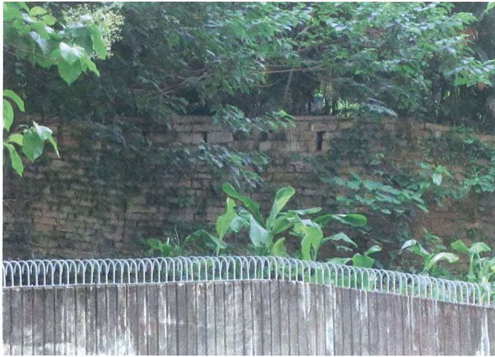
E.5 Corner of historic fortified, defensive squared rubble masonry wall with loopholes for firing can be seen from Cotton Tree Drive above Fire Station compound. Flagstaff House garden area is behind.
