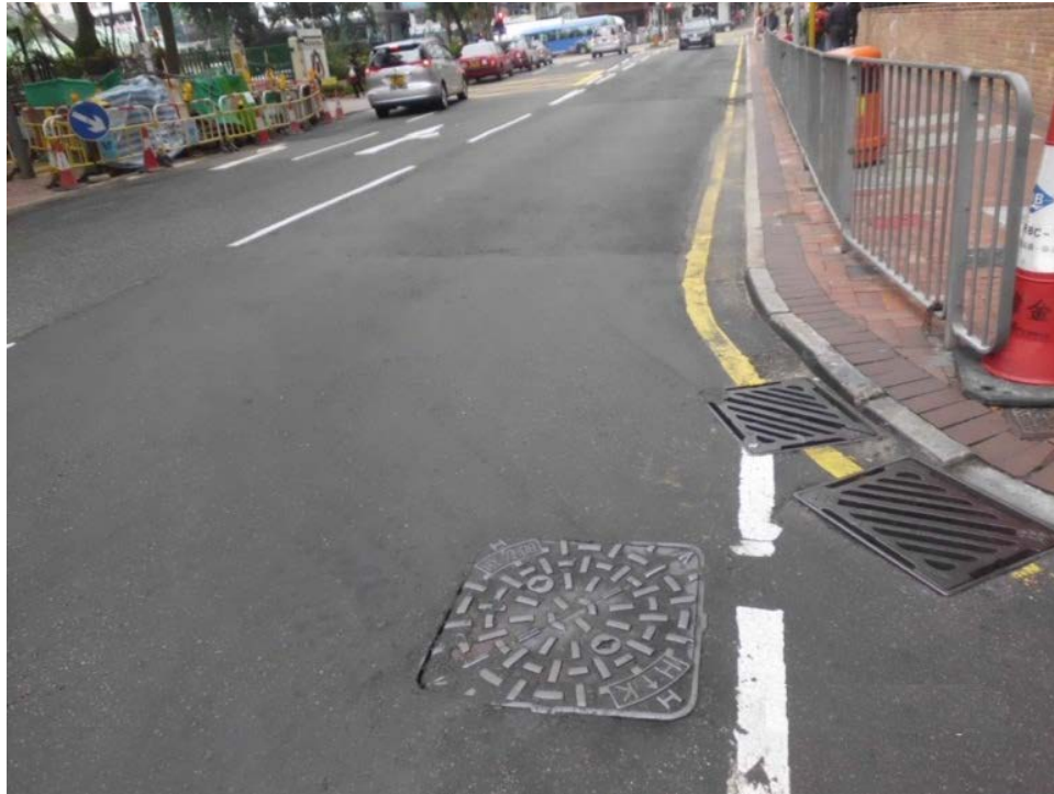
Figure 3: Photo of road resurfaced by thermal patcher
