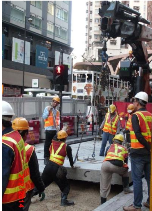
Figure 5: Placing precast concrete panel on-site
