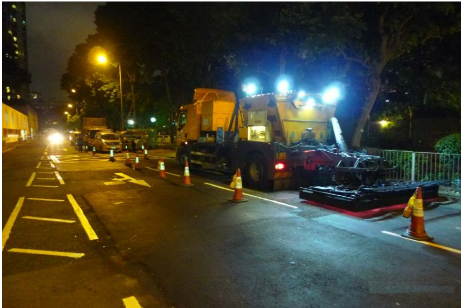
Figure 2: Pavement resurfacing by thermal patcher
