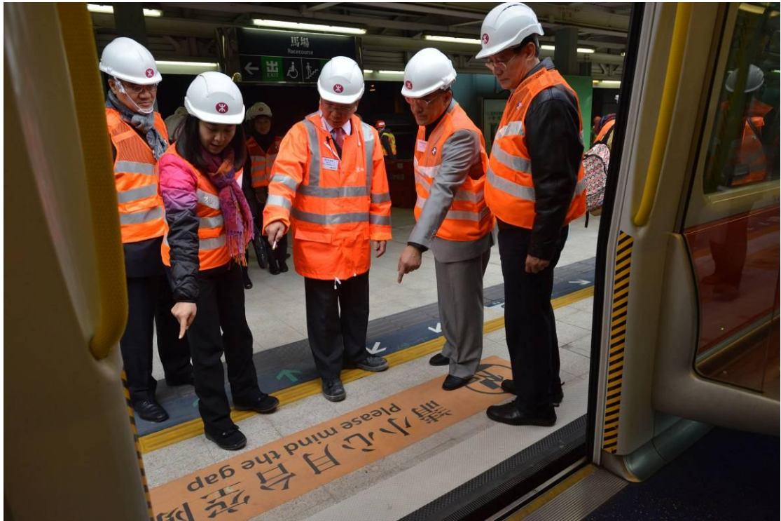
LegCo Members visit the Racecourse Station to observe the platform modification works.
