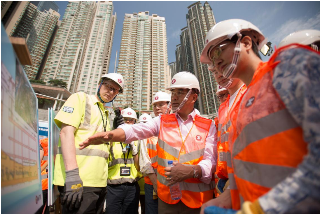
Members receive a briefing from the representatives of the MTR Corporation Limited on the latest progress of the works.
