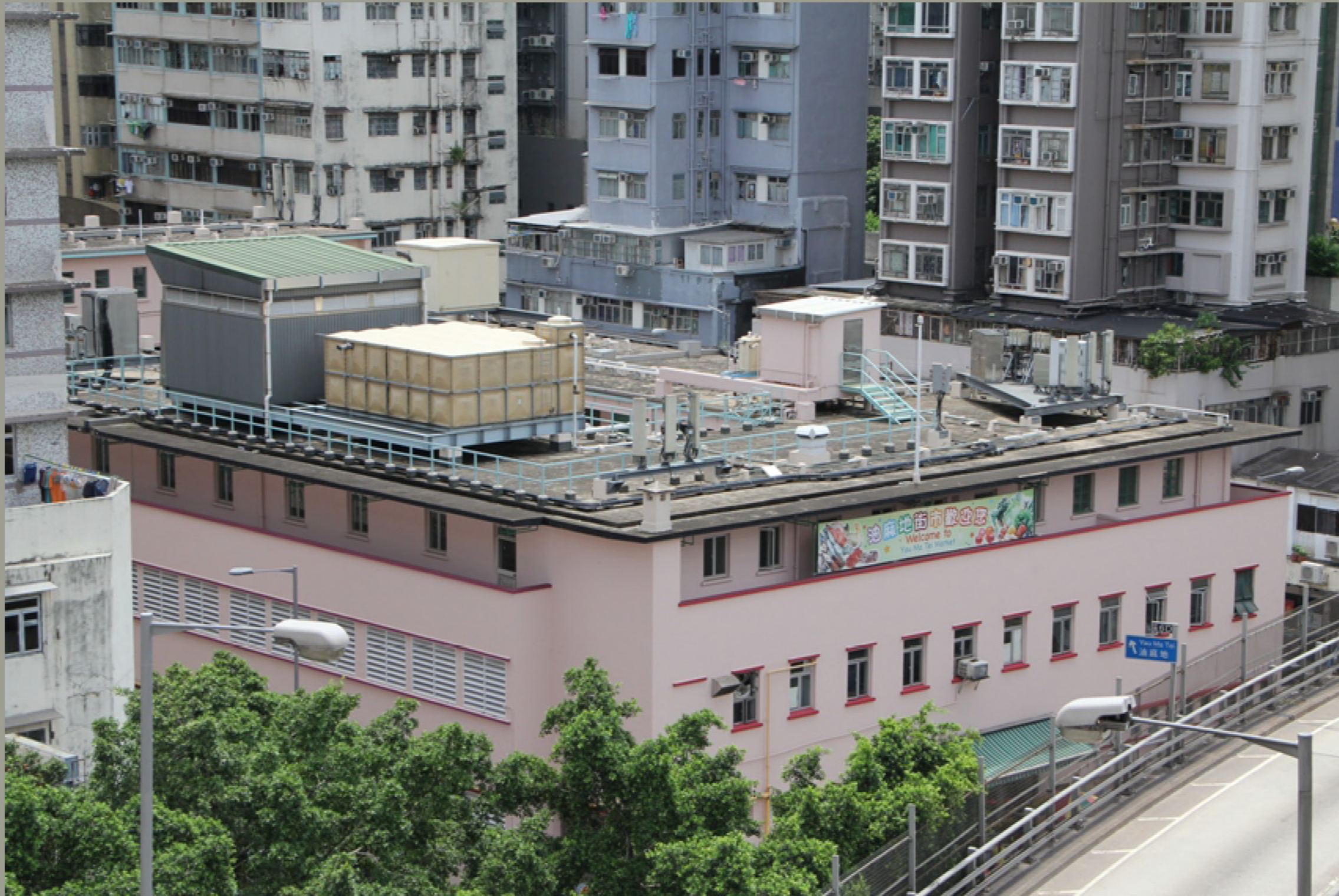
EXISTING STRUCTURE ON ROOFTOP
