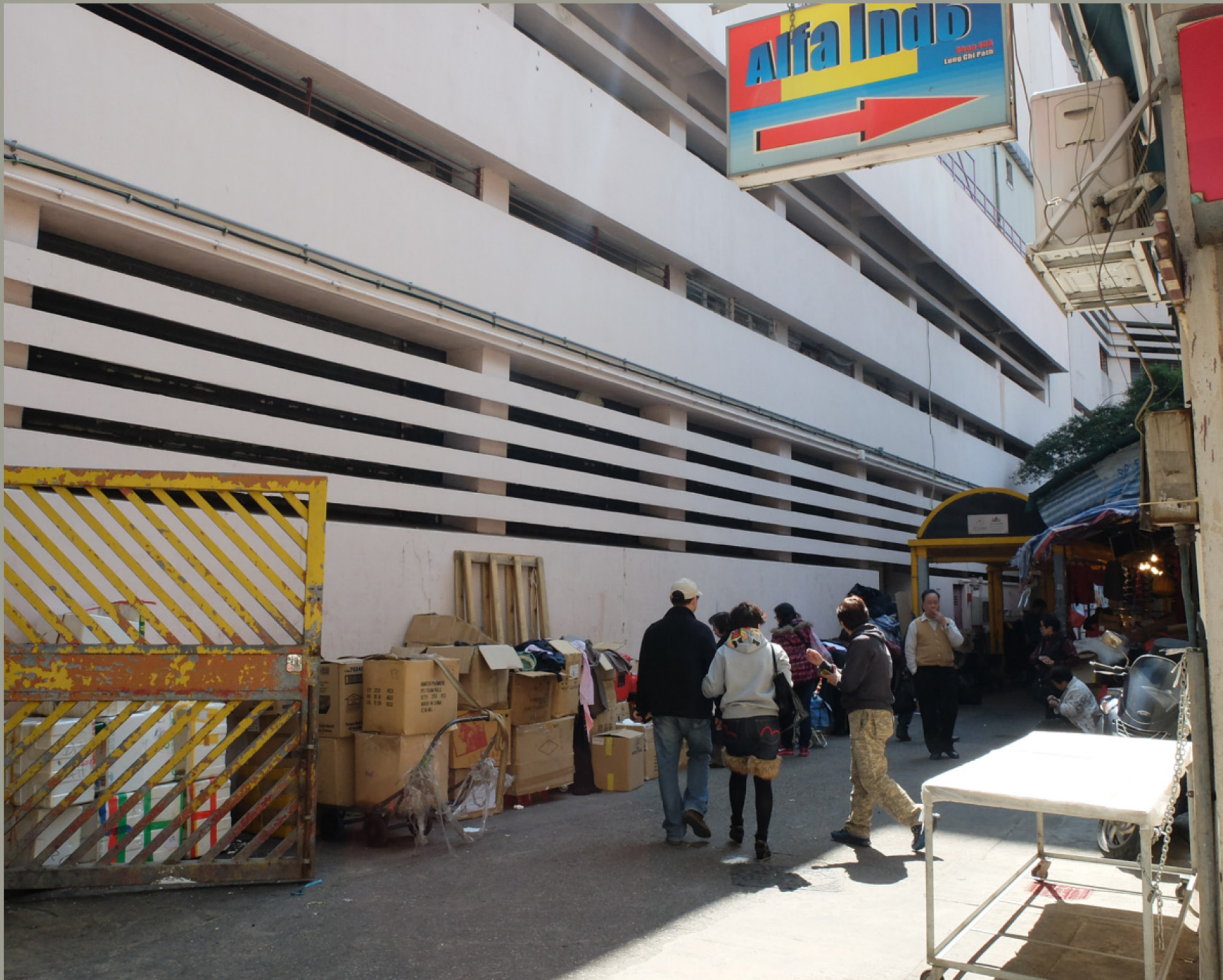
FACADE FACING KAM CHI PATH
