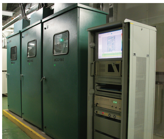
Optical Sensing Ltd's Distributed Temperature Sensing System was installed at Energy Tower 1 for real-time temperature monitoring
