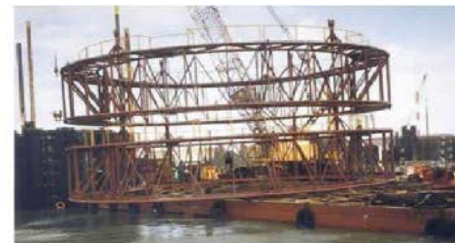
D. TEMPLATE USED TO STABILIZE CIRCULAR CELL 穩定圓環式圍堰的模板
