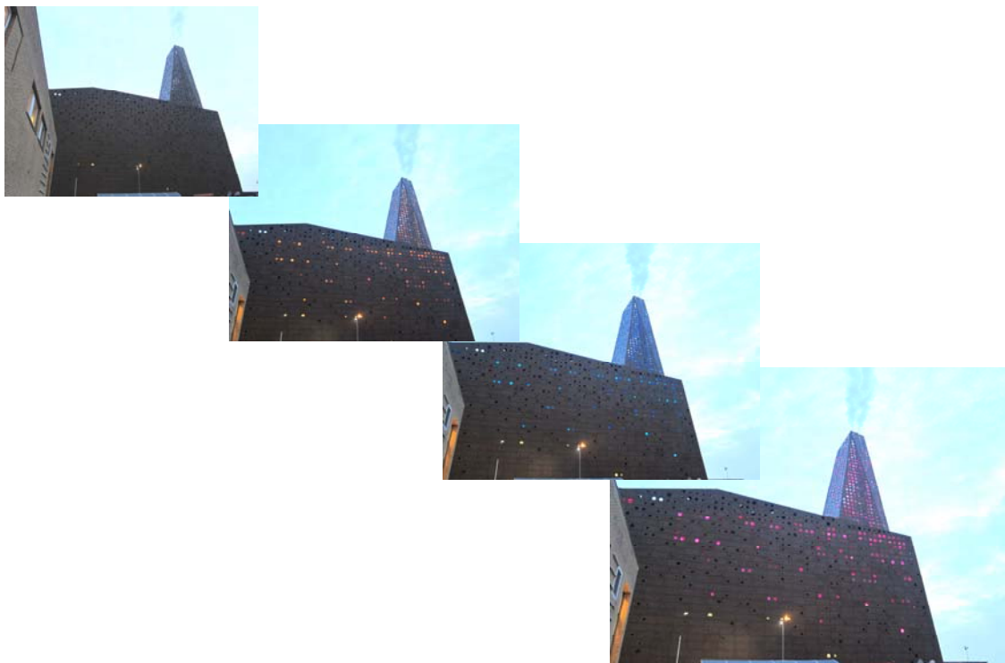
Circular openings in the building's aluminium facade serve to transform the station into a beacon at night, when light from the facility shines through the exterior
