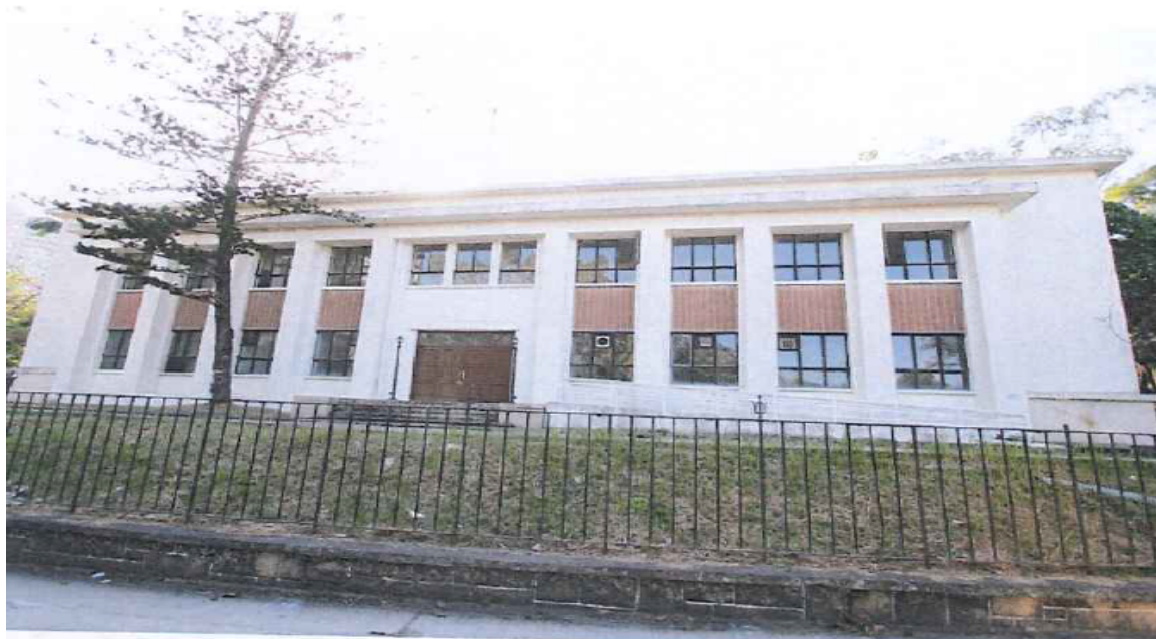
Existing Conditions of Former Fanling Magistracy 前粉嶺裁判法院的現貌
