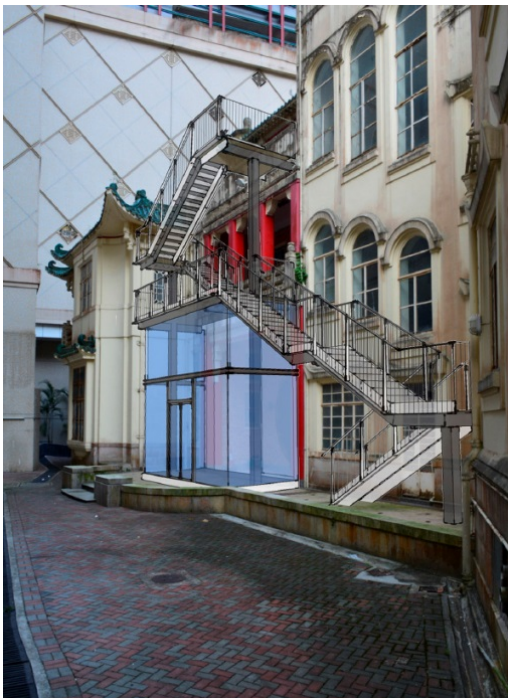
New Rear Staircase 新建後樓梯
