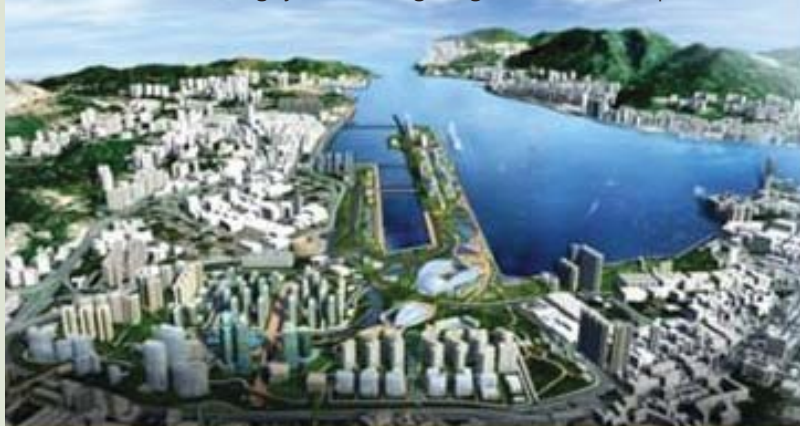
The first district cooling system in Hong Kong at Kai Tak Development
