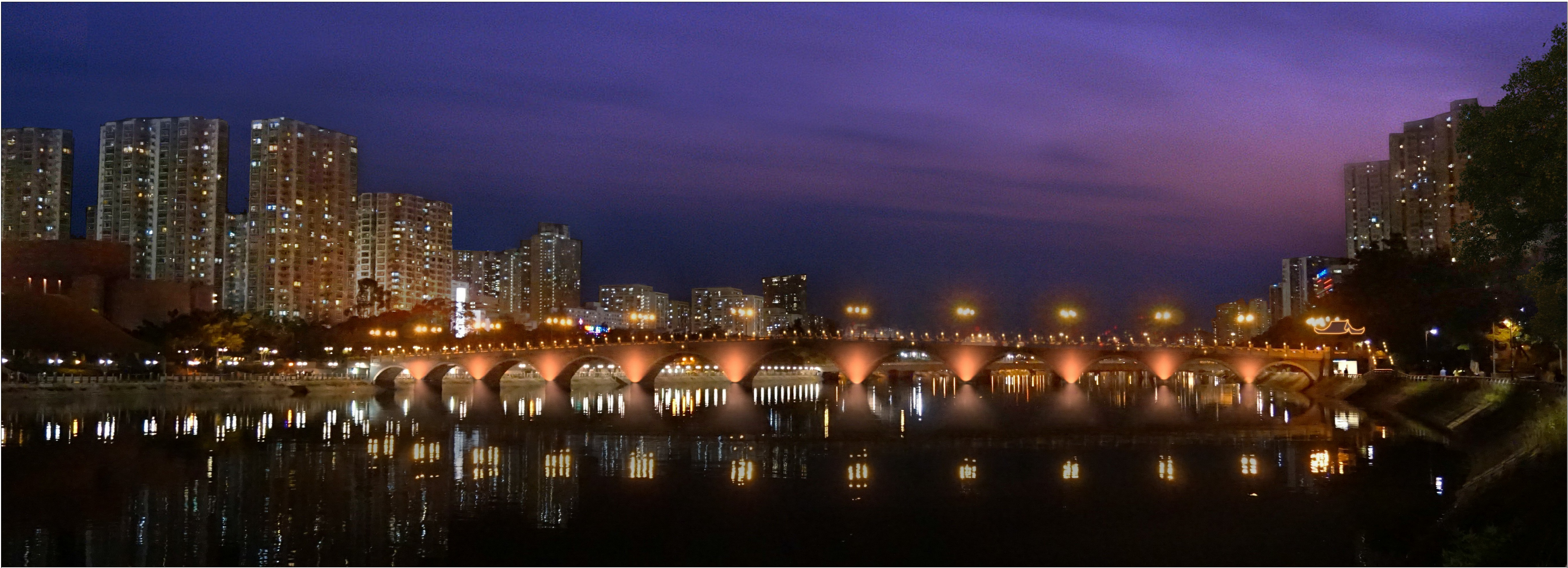
瀝源橋 LEK YUEN BRIDGE
