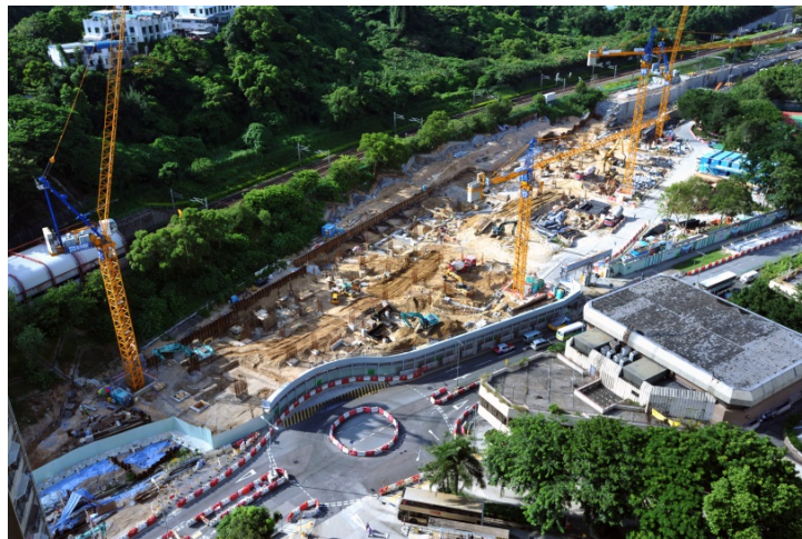
Hin Keng Station construction site
