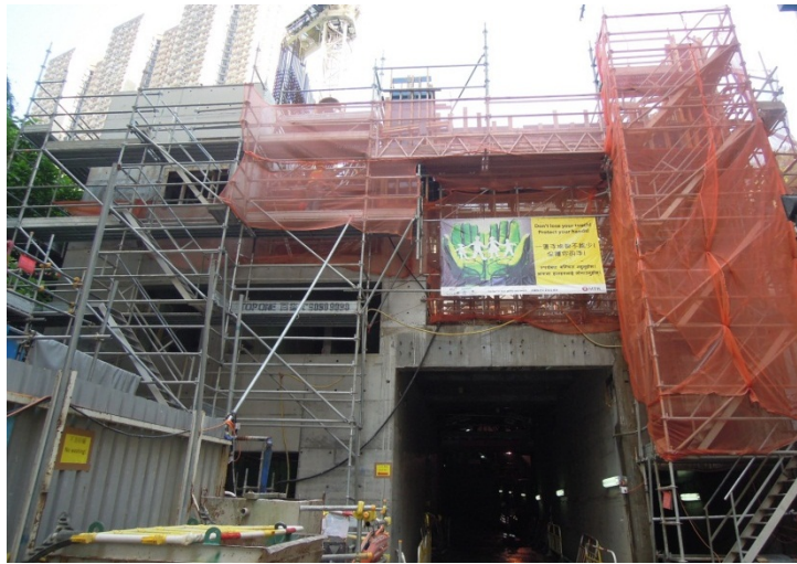
Structural works of Lei Tung Station Entrance A
