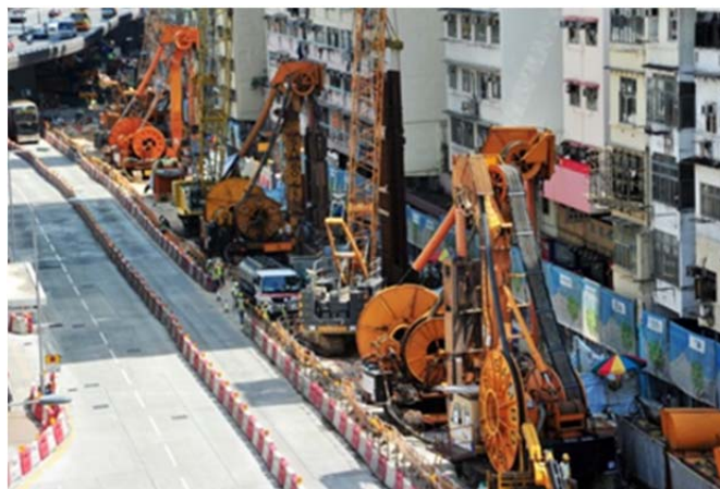
Ma Tau Wai Station construction site
