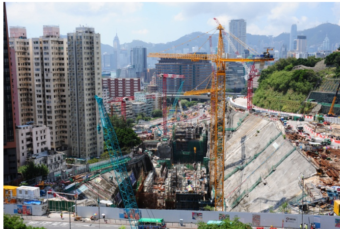
Structural works of Ho Man Tin Station
