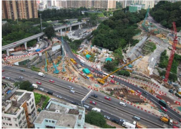
Piling works at the north of Hung Hom Station
