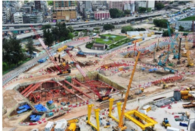
To Kwa Wan Station construction site
