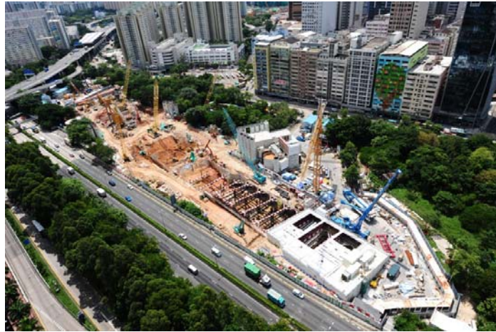
Diamond Hill Station Extension construction site
