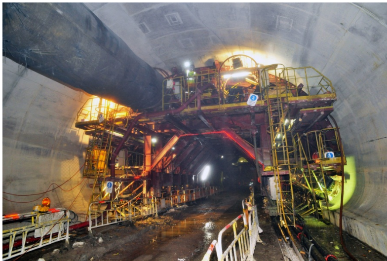
Nam Fung Tunnel permanent lining works
