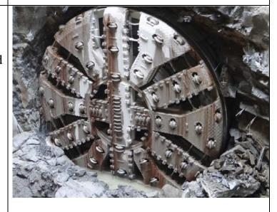
Re-assembly of TBM of Shek Kong southern section for the excavation of the northbound tunnel (823A)
