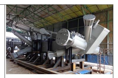
Large-scale temporary support structure for construction of the Terminus roof structure (810A)
