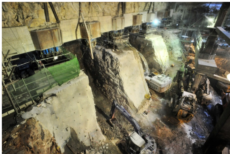
Island Line tunnel underpinning works at Admiralty Station
