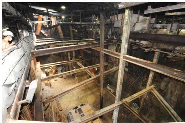
Excavation of the East and West Concourses of Whampoa Station
