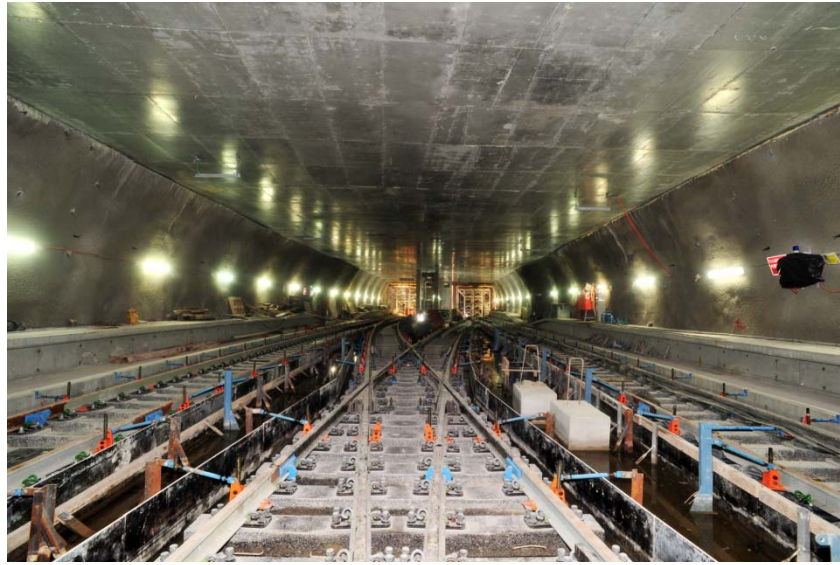
Track-laying works in the tunnel on Ap Lei Chau
