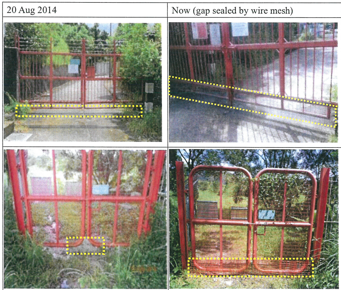
Figure 8. Improvement work performed on the gaps of two gates.
