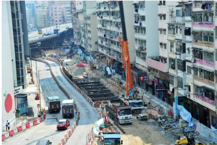
Ma Tau Wai Station construction site
