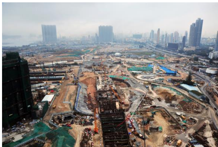
Kai Tak Station construction site
