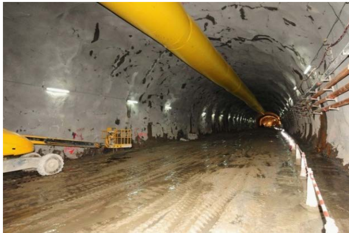
Tunnel construction inside the Lion Rock
