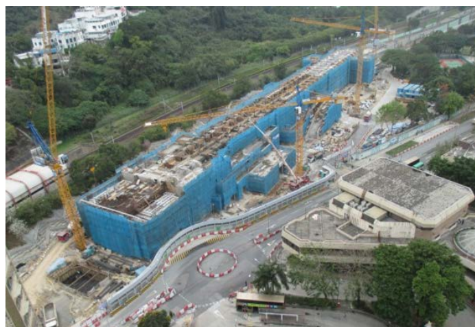
Hin Keng Station construction site
