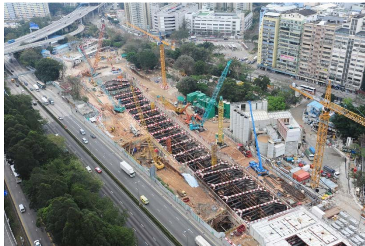
Diamond Hill Station Extension construction site
