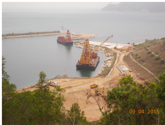
Casting Yard for IMT units
