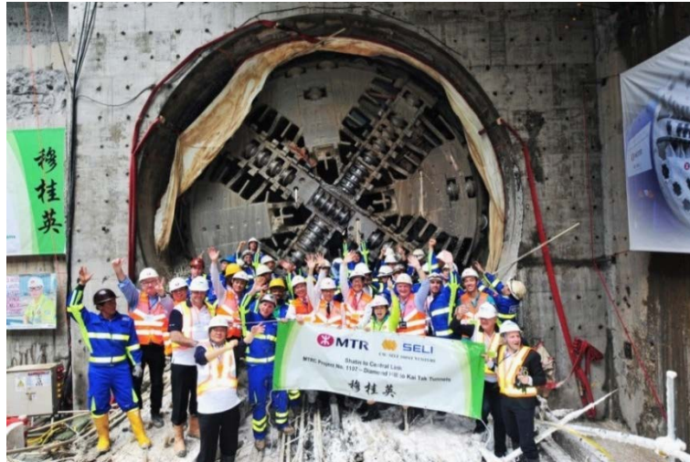
Breakthrough of the up-track tunnel from Kai Tak to Diamond Hill
