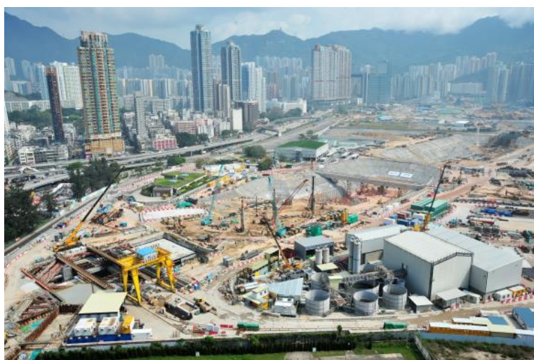
To Kwa Wan Station construction site
