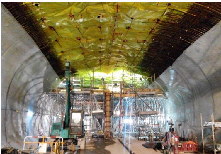
Nam Fung Tunnel permanent lining works
