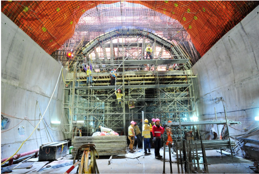
Structural works of Lei Tung Station entrance at Lei Tung Estate
