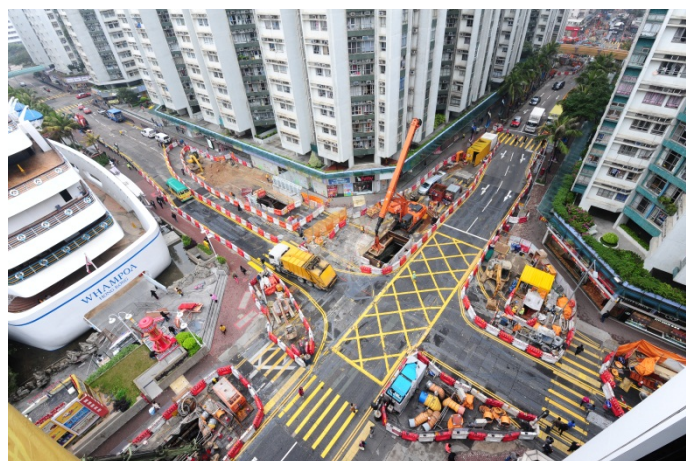
Construction sites of the East concourse of Whampoa Station
