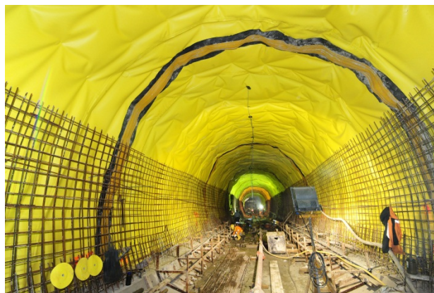
Lining works of Whampoa Station overrun tunnel
