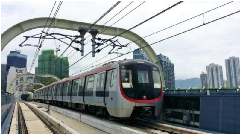
Train testing on the running track between Wong Chuk Hang Station and South Horizons Station has commenced
