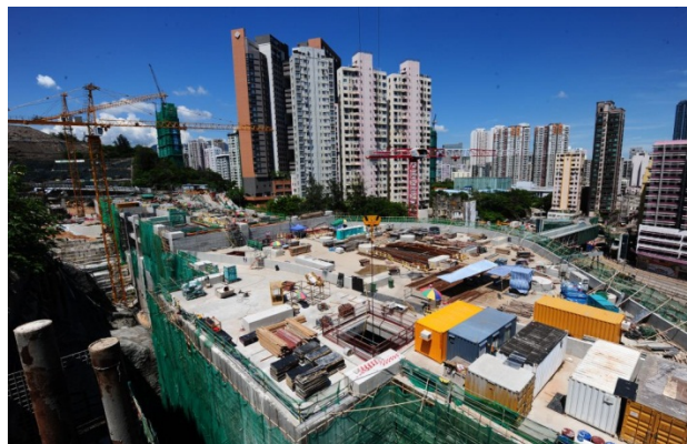
Ho Man Tin Station has been topped out.
