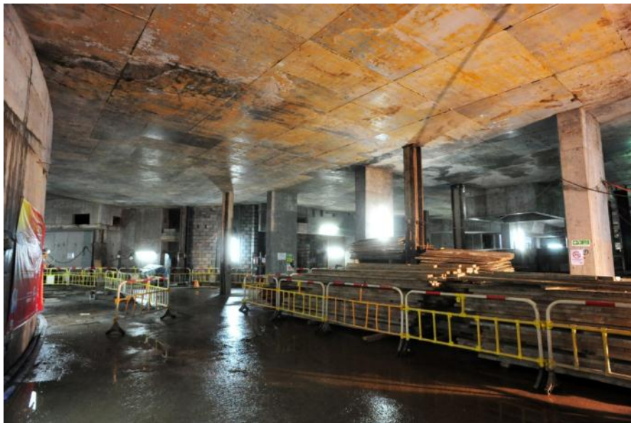
Station structural works under the temporary traffic deck at South Horizons
