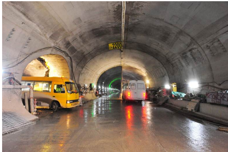
Nam Fung Tunnel permanent lining works are substantially completed
