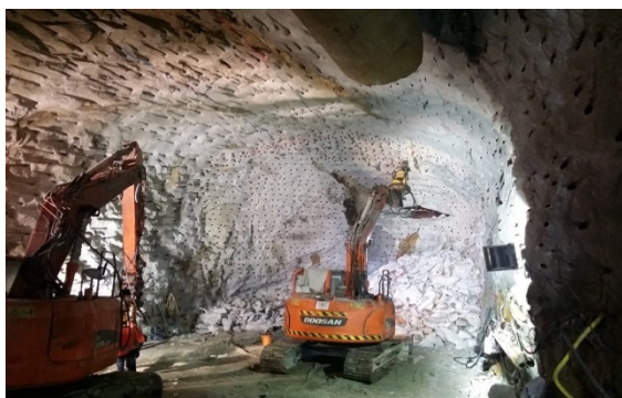
Excavation for Platform Tunnel of Whampoa Station
