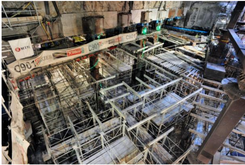
Underpinning works for Island Line tunnel at Admiralty Station
