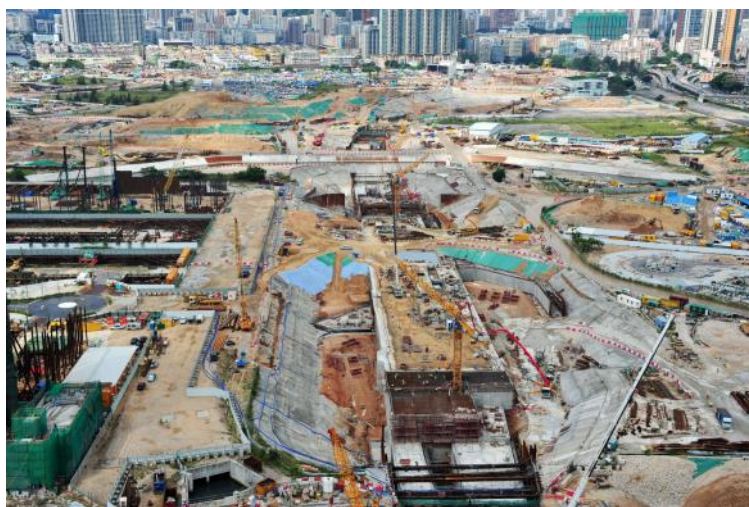
Kai Tak Station construction site
