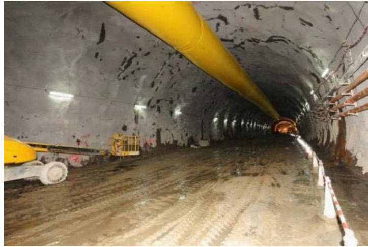
Tunnel construction inside the Lion Rock
