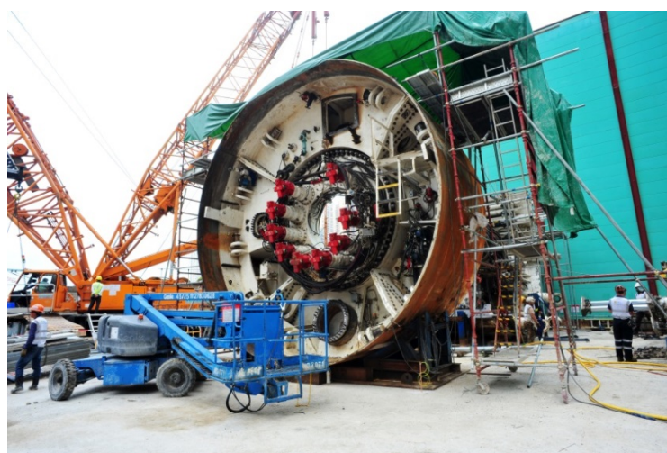
TBM reassembling works at Kai Tak works site
