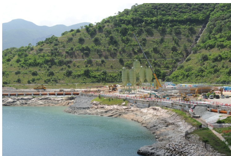
Casting Yard for IMT units
