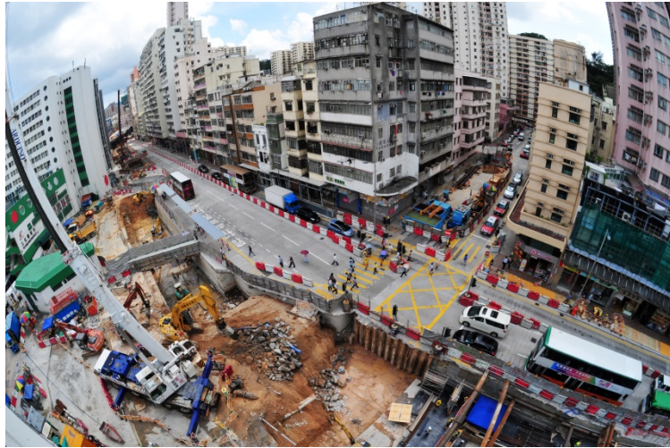
Ma Tau Wai Station construction site
