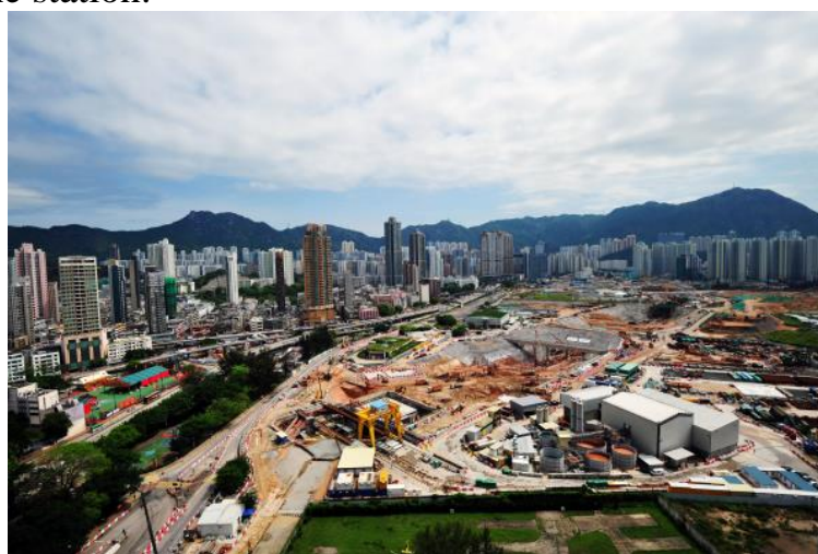
To Kwa Wan Station construction site
