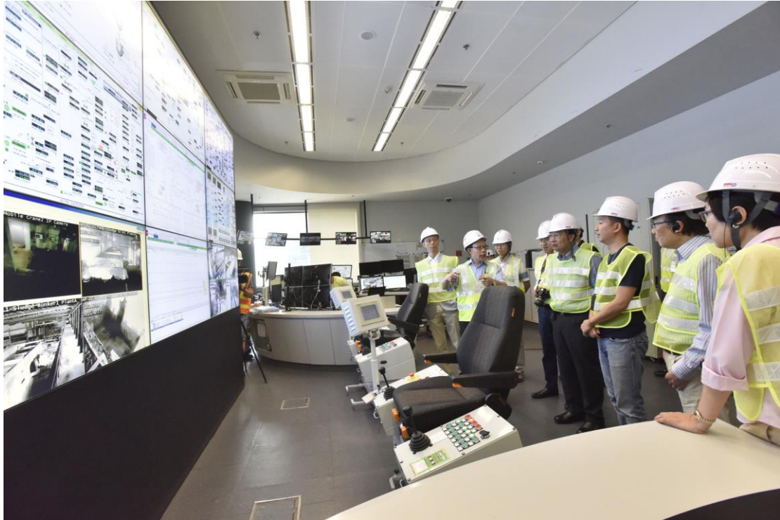
Members of the Legislative Council visit the Central Control Room in the Sludge Treatment Facility in Tuen Mun.
