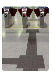
Tactile guide paths are installed at all stations and Light Rail stops. For the convenience of visually impaired passengers, tactile guide paths in station concourses lead to an exit gate with an audible device providing audible Octopus readings.
