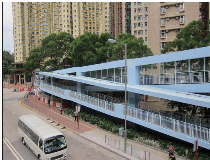
A ramp of a footbridge in Wong Tai Sin
