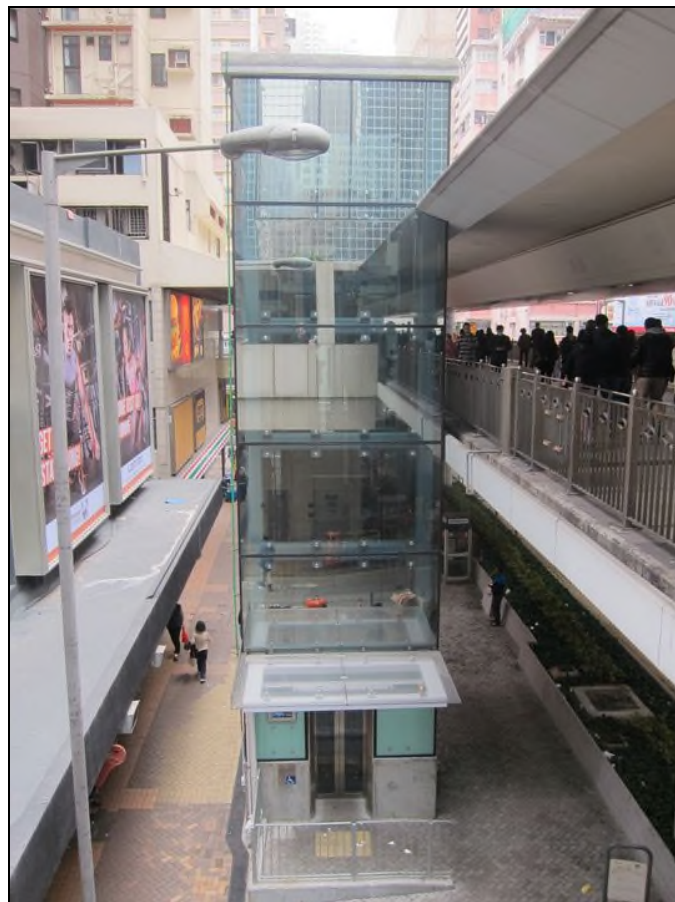
A passenger lift for a footbridge in Wan Chai
