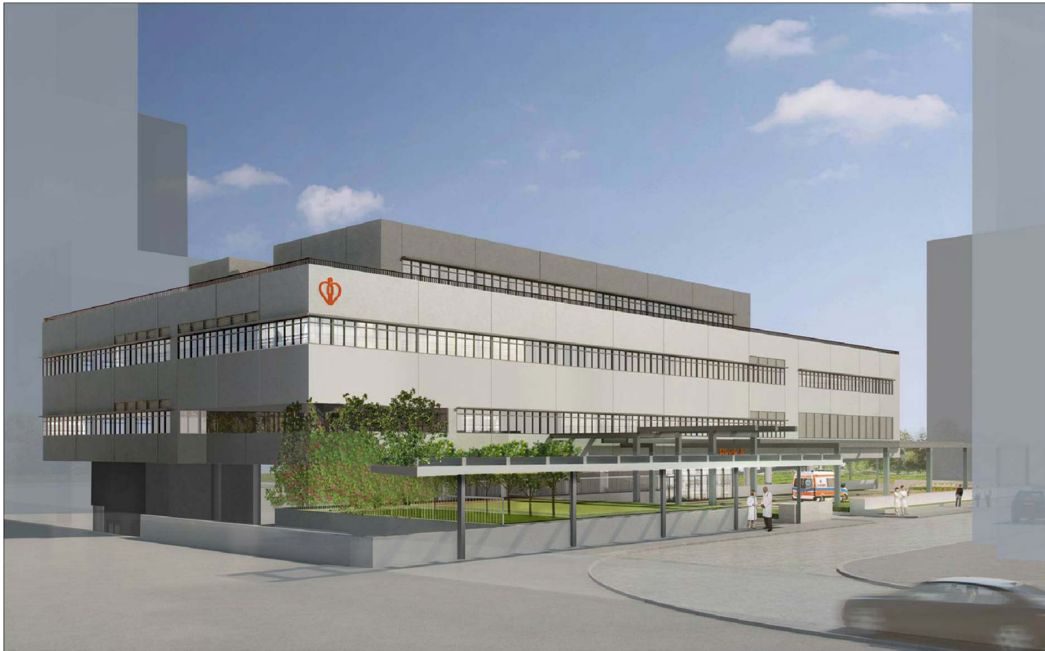
從南面望向調遷大樓的構思透視圖 PERSPECTIVE VIEW FROM SOUTHERN DIRECTION (ARTIST'S IMPRESSION)
