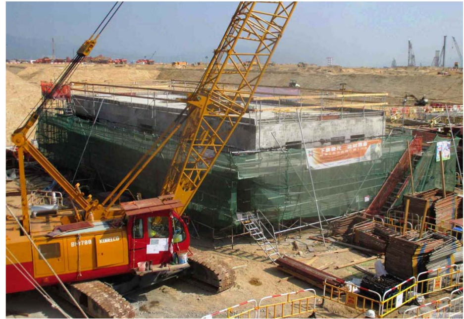
The external structural works of the Weigh Station have commenced
