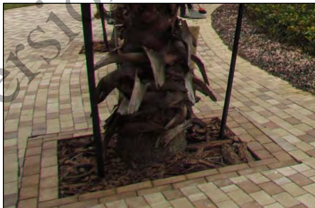
Fig. 9 Permeable paver blocks on sand base
