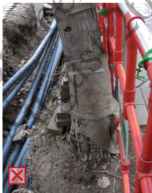
Photo 9 - Excavation within tree protection zone will cause significant damage to root system
