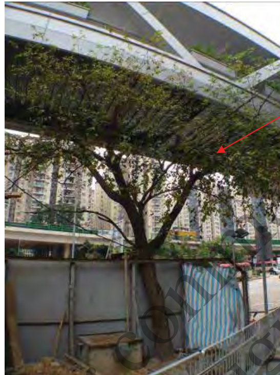
Tree growing under a footbridge with restricted headroom
