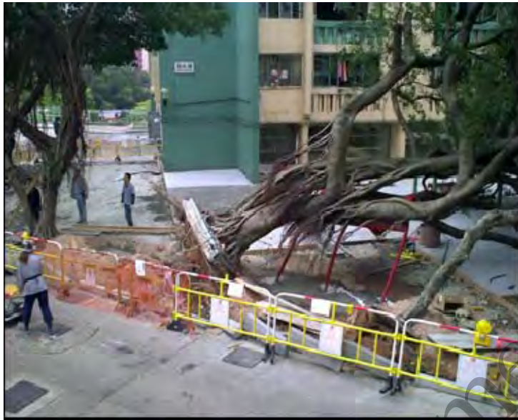
Fig. 3 Ficus microcarpa collapsed during repaving
