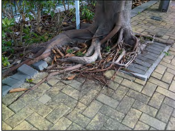
Fig. 8 Trees with aggressive roots in confined tree pits
