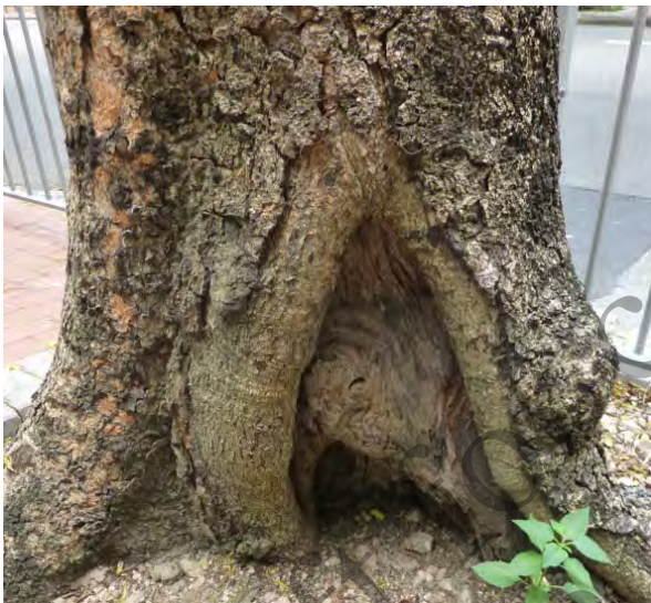
Photo 2.8 - Wood decay/cavity at basal area/root flare
