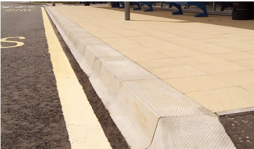
Bus stop with 160mm high kerb (source: Kassel)
