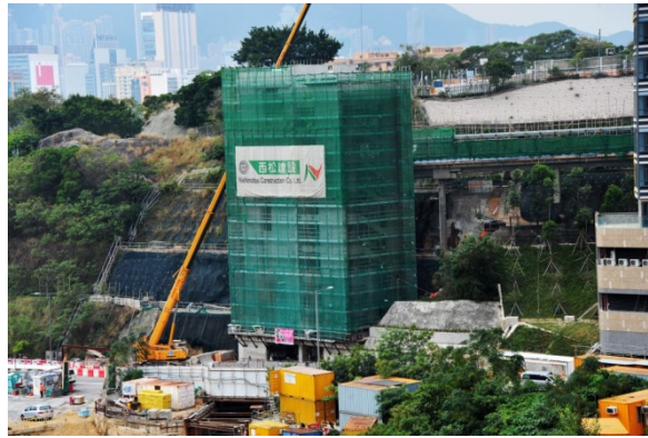
Structure of the lift tower at Chung Hau Street is completed
