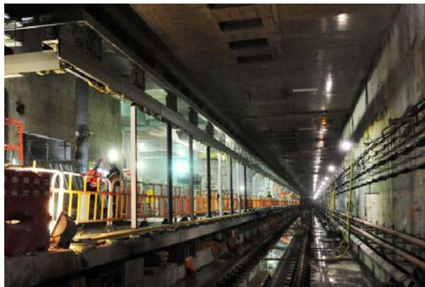
Overhead lines installation works underneath Tak On Street
