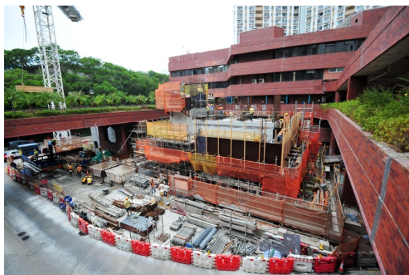
Above-ground structural works of Lei Tung Station Entrance B
