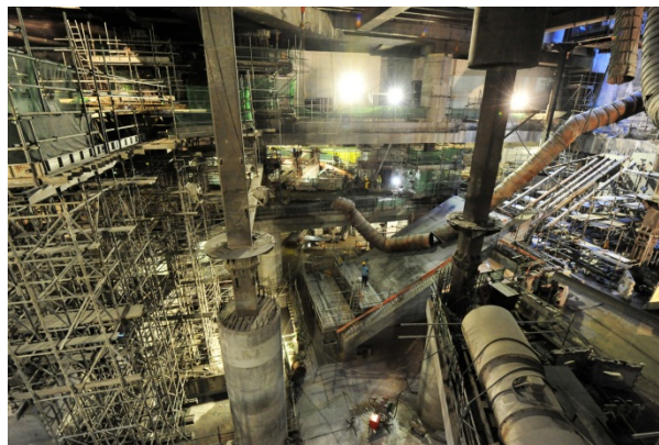
Structural works continue for the Admiralty Station extension
