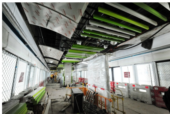
Fitting-out and E&M works at South Horizons Station
