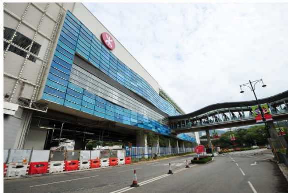
Structural works of the covered footbridge connecting Ocean Park Station to the theme park's entrance are completed
