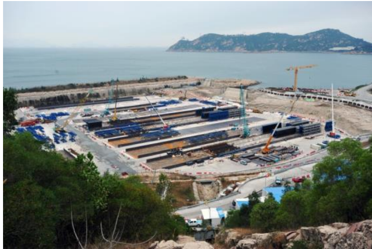
Casting yard of IMT pre-cast units
