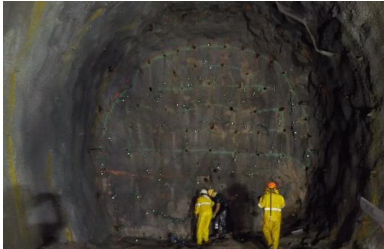
Excavation of ventilation tunnel in progress at Ma Chai Hang
