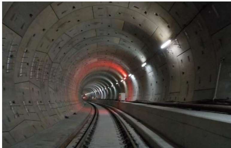
Track-laying at DIH up-track tunnel
