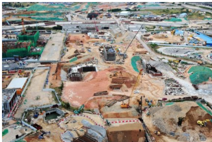
Kai Tak Station Construction Site
