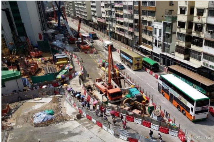
Construction site of Ma Tau Wai Station
