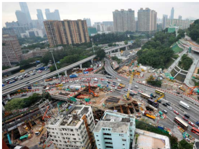
Tunnel excavation under Chatham Road North and near Winslow Street
