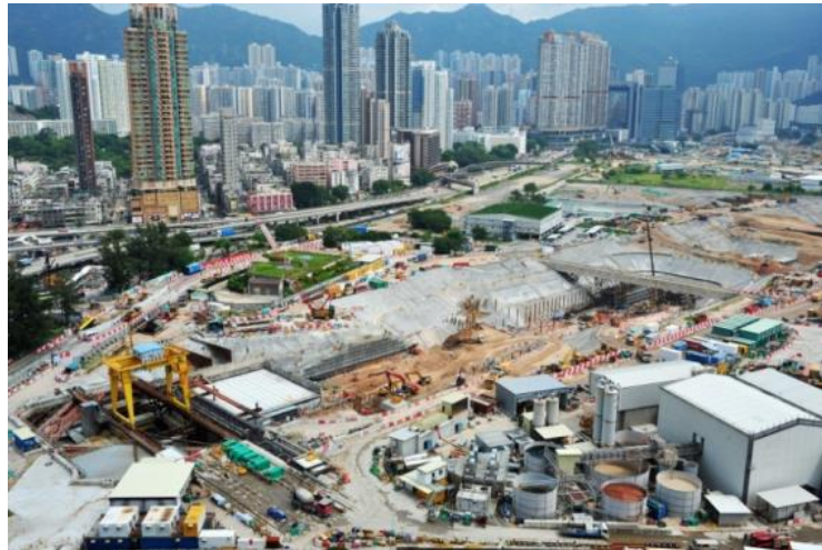
Construction site of To Kwa Wan Station
