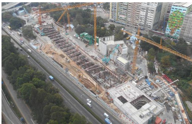
Expansion works of Diamond Hill Station
