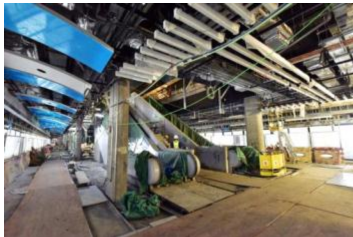
Fitting-out and E&M works at Admiralty Station are underway
