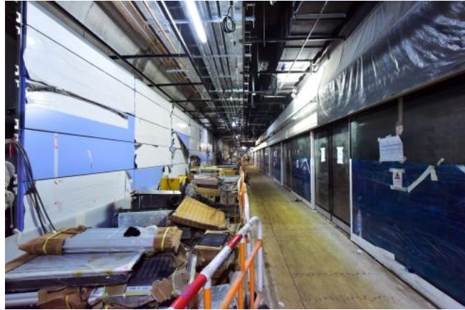
E&M equipment are being installed at the Whampoa station platform.
