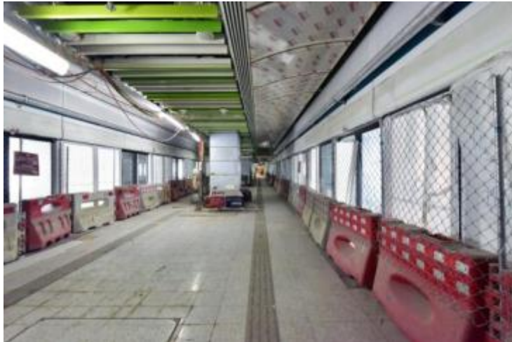
Fitting-out and E&M works at South Horizons Station are underway
