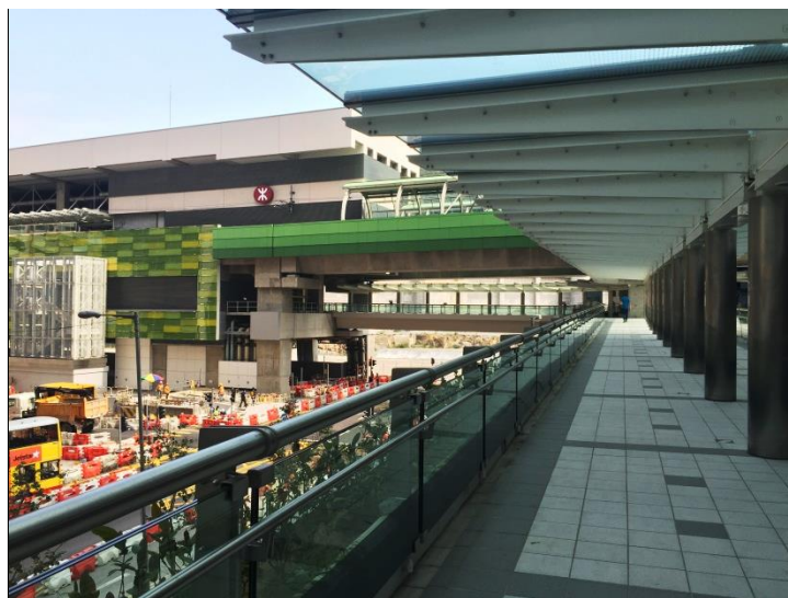
A covered footbridge connecting Wong Chuk Hang Station to the adjacent area was opened for public use
