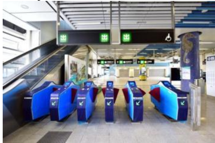
Testing for station facilities and various systems at Ocean Park Station and Wong Chuk Hang Station is underway
