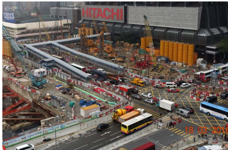
Exhibition Station Construction Site
