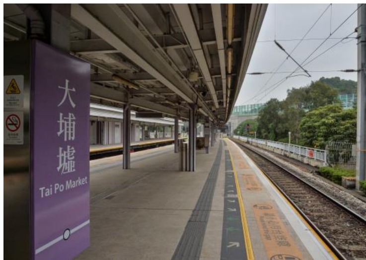
Platform strengthening works along EAL
