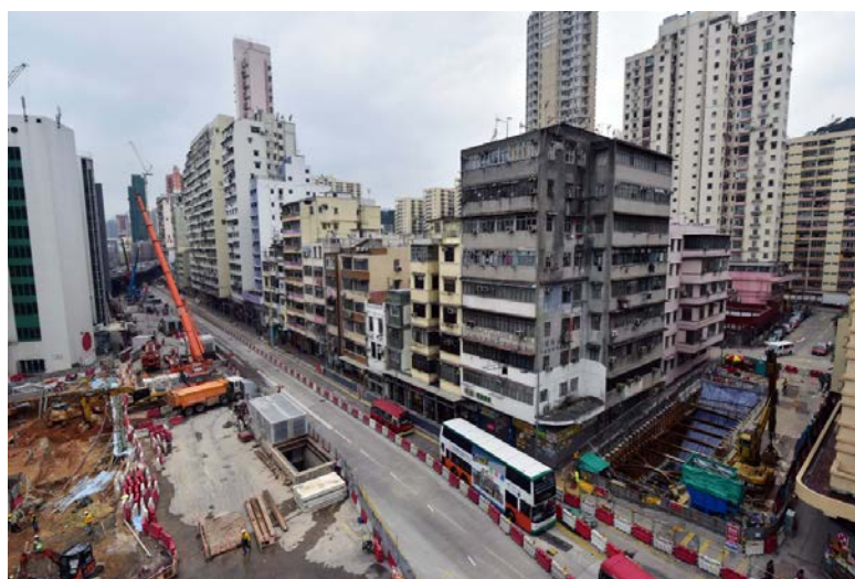
Construction site of Ma Tau Wai Station
