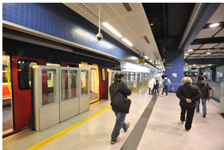
Retrofitting works of APGs at Tai Wai Station were completed
