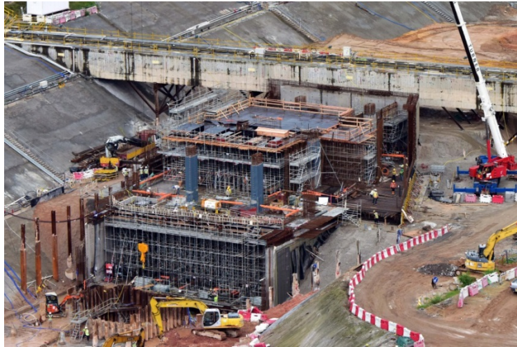
Structural works for To Kwa Wan Station
