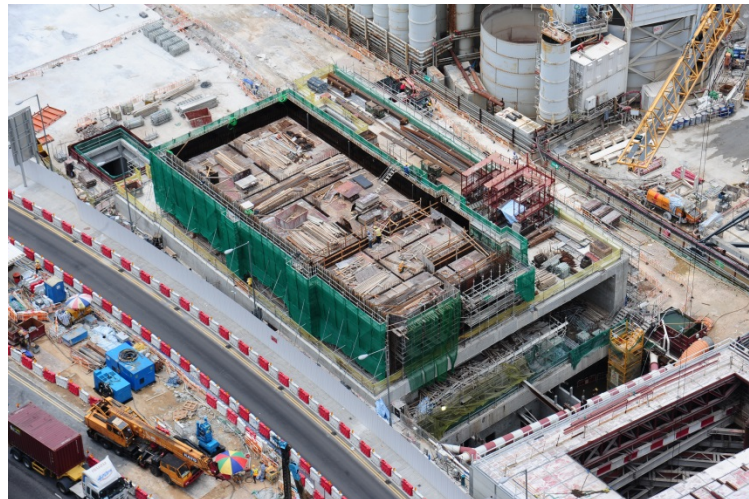
Expansion works for Diamond Hill Station
