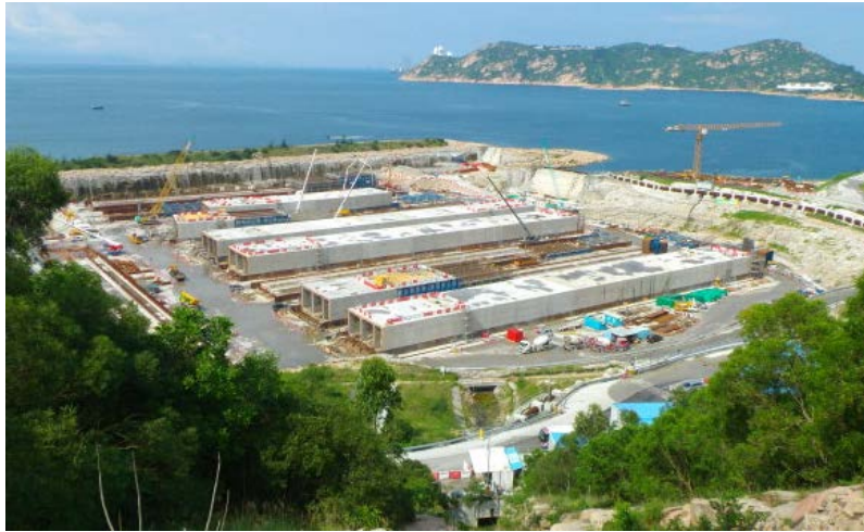
Casting yard of IMT pre-cast units
