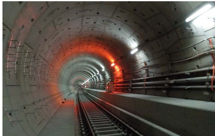
Track-laying at Diamond Hill up-track tunnel
