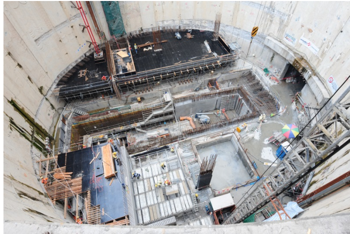
Structural works for the ventilation shaft at Ma Chai Hang
