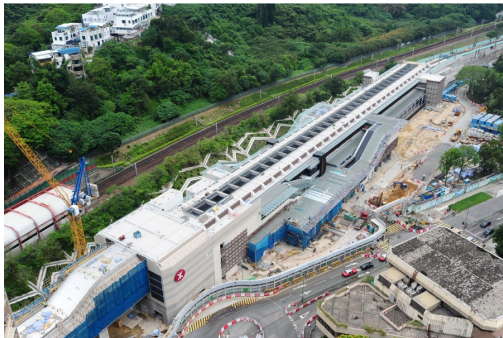
Hin Keng Station and part of the viaduct
