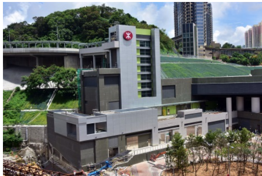
External finishing works of Ho Man Tin Station is substantially completed.
