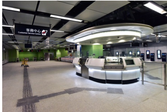
Station facilities at Ho Man Tin station are installed.
