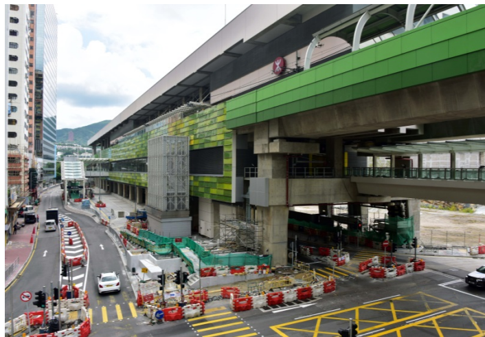
The PTF at Wong Chuk Hang Station were opened in June 2016
