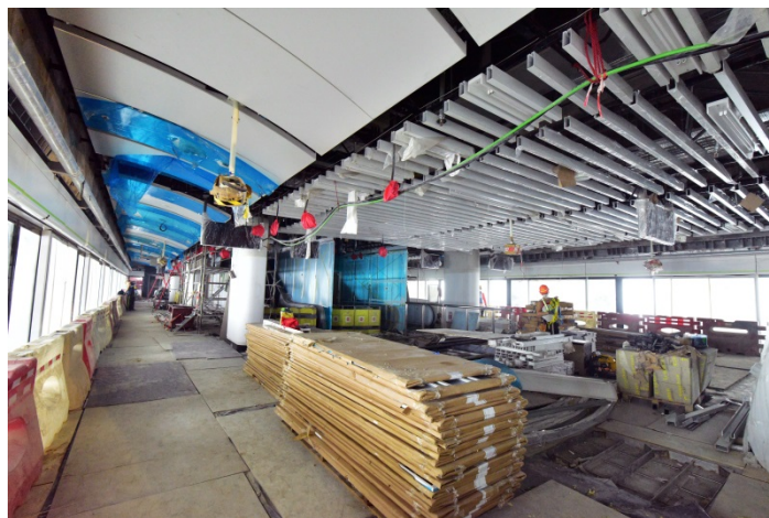
Fitting-out and E&M works at the SIL(E) platform level are underway
