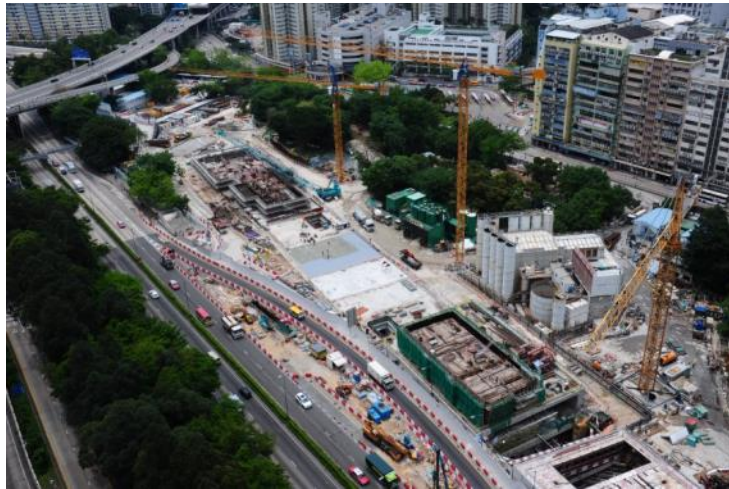
Expansion works for Diamond Hill Station
