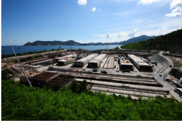
Casting yard of IMT pre-cast units
