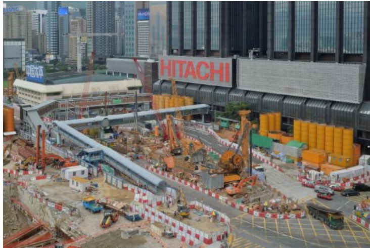
Exhibition Station Construction Site
