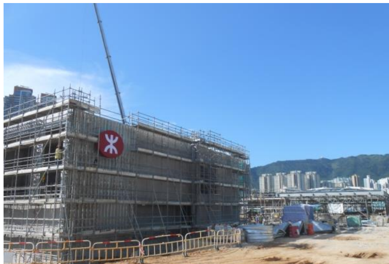
Entrance D and Ventilation Shaft Building at Kai Tak Station
