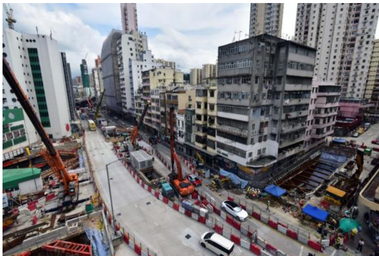
Construction site of Ma Tau Wai Station
