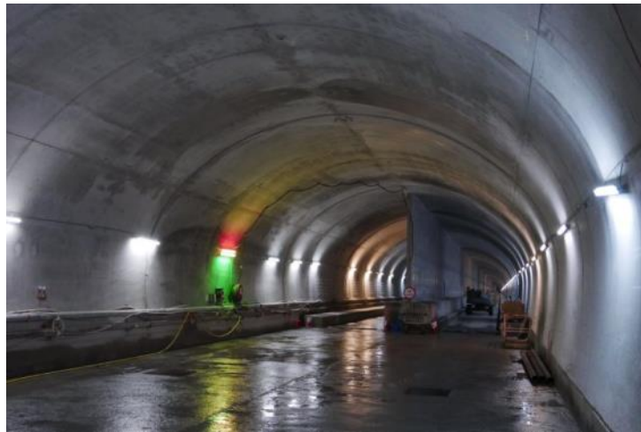
Tunnel inside Lion Rock
