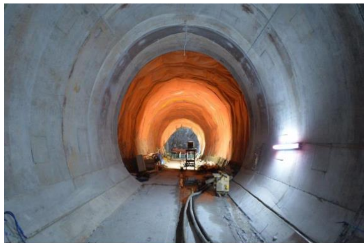
Tunnel lining works for the ventilation tunnel at Ma Chai Hang
