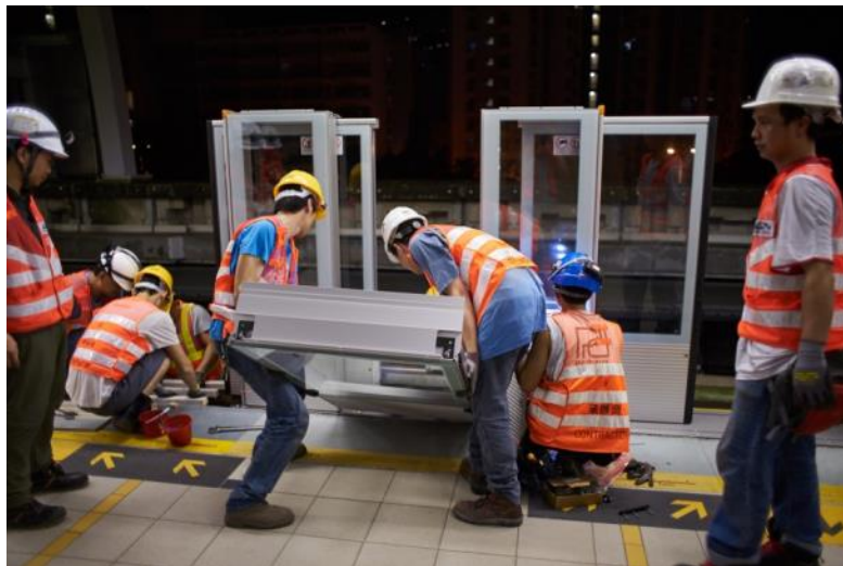
Retrofitting works of APGs
