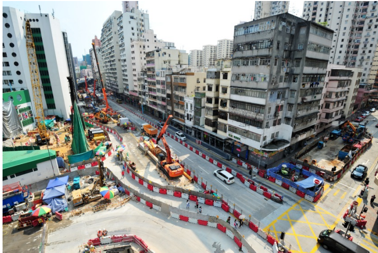
Construction site of Ma Tau Wai Station
