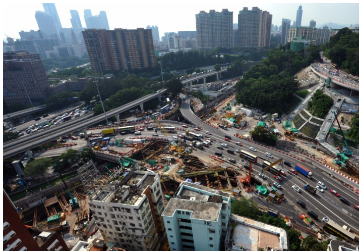
Tunnel excavation under Chatham Road North and near Winslow Street
