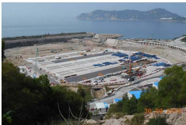
Casting Yard of IMT Pre-cast Units
