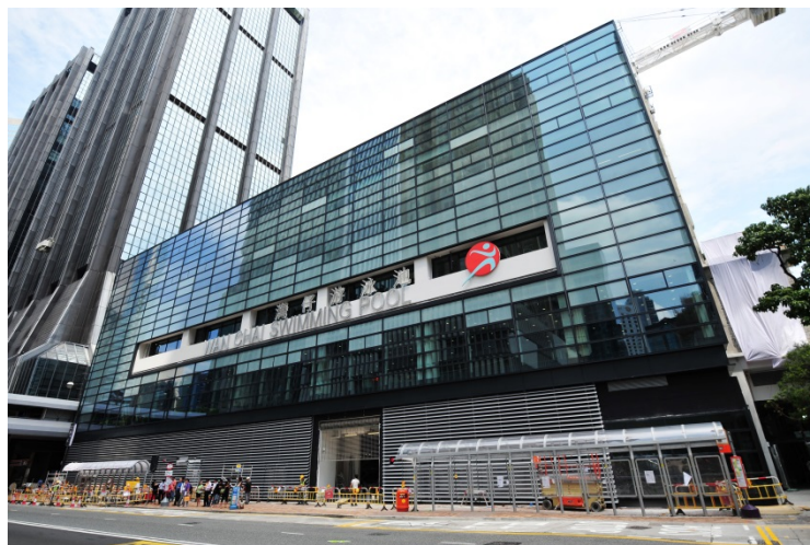
The reprovisioned Wan Chai Swimming Pool is substantially completed
