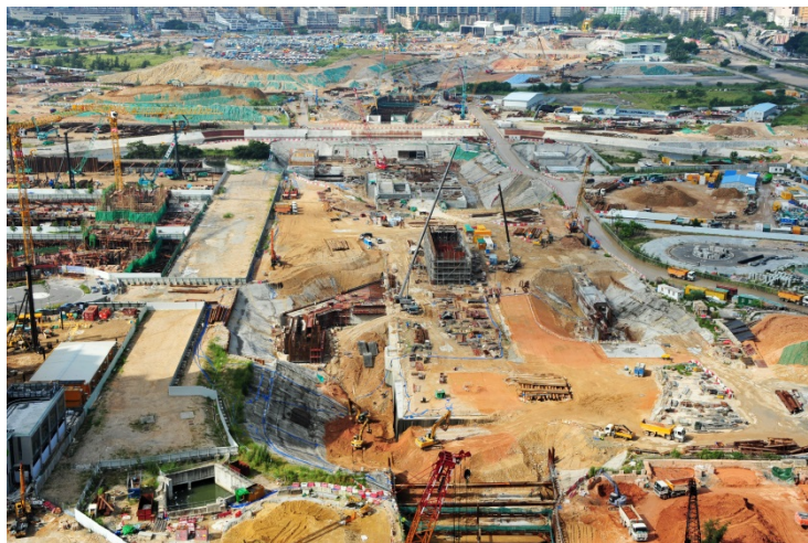
Kai Tak Station Construction Site
