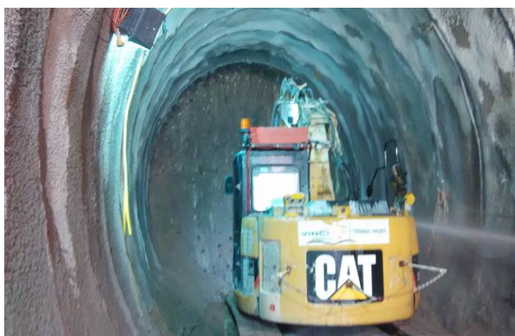
Excavation of ventilation tunnel in progress at Ma Chai Hang
