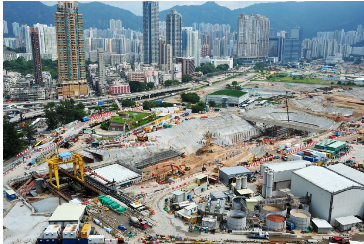
Construction site of To Kwa Wan Station
