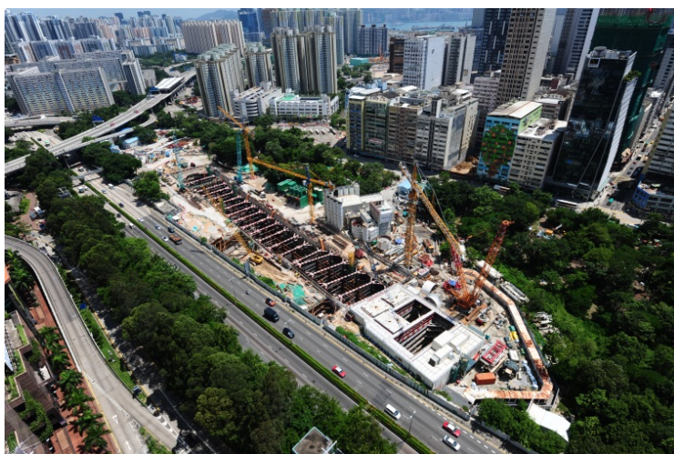
Expansion works of Diamond Hill Station
