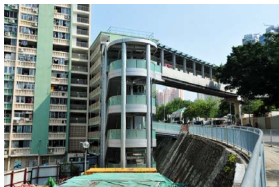
Pedestrian facilities connecting Oi Man Estate and Ho Man Tin Estate were completed
