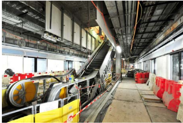
Fitting-out and E&M works at Lei Tung Station
