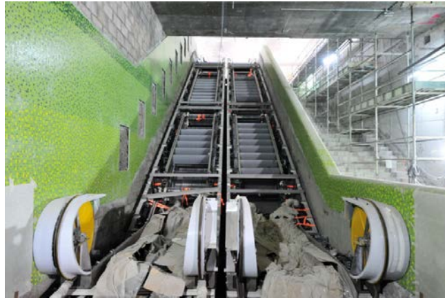
E&M Installation works at Ho Man Tin Station
