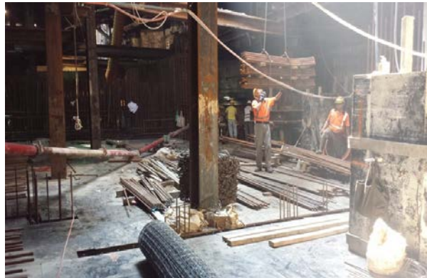
Structural works at East Concourse of Whampoa Station
