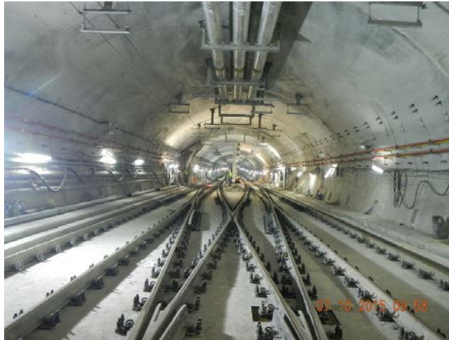
Track-laying works underneath Tak Man Street
