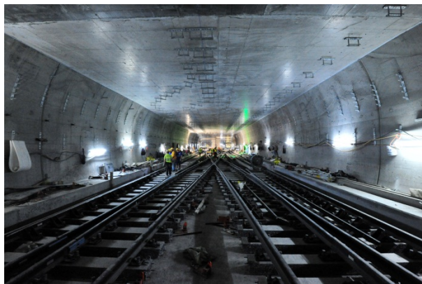
Nam Fung Tunnel permanent lining works have been completed
