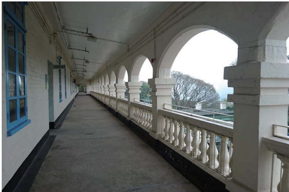
Tuscan-style columns, Classical urn-shaped balustrades and granite coping stones of the verandah.
