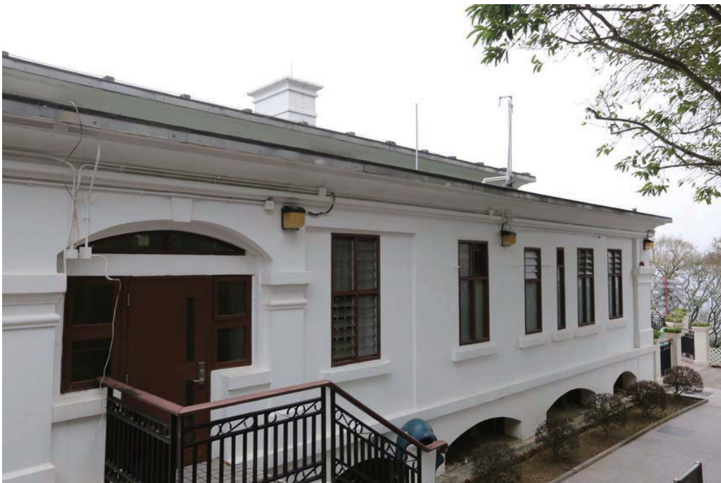
The two-step flat roof converted from the original pitched "Jack-Roof".
