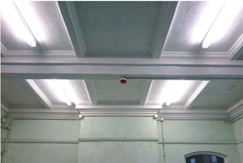
Classical plaster mouldings to the ceiling cornices and picture rails of the old dining room.
