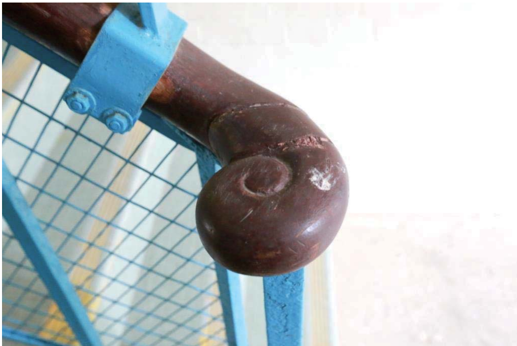
The handrail scroll of an internal staircase.
