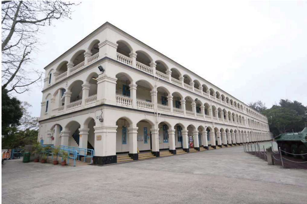
The east facade featuring the long open arched, colonnaded and balustraded verandahs.
