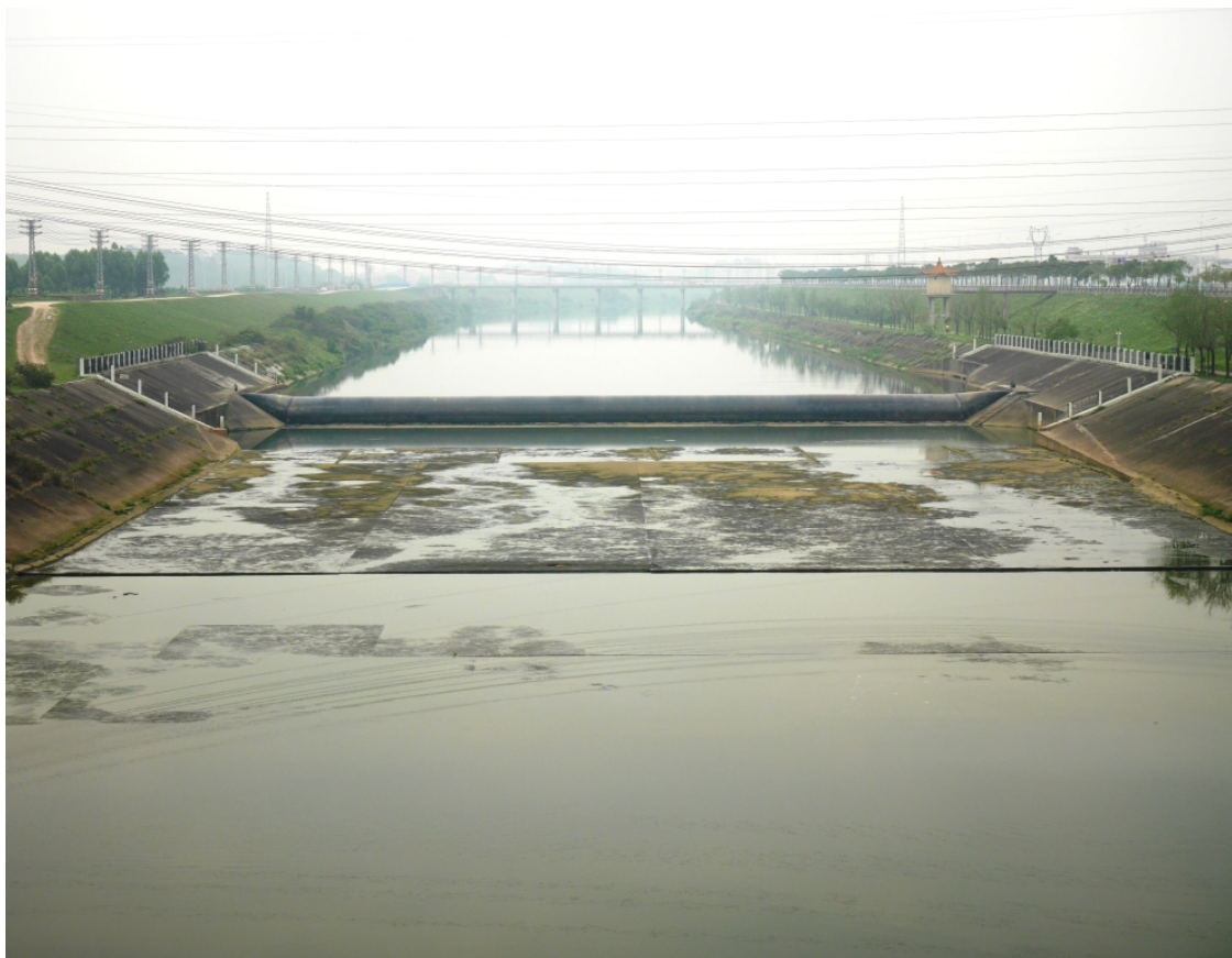
Rubber dam on the Shima River prevents contaminated water from flowing into Dongjiang
