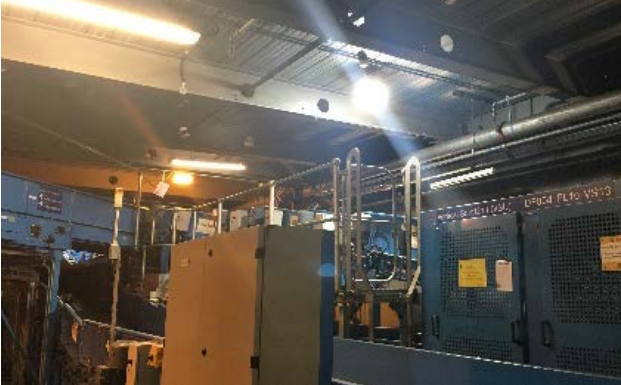
LED Light Replacement
