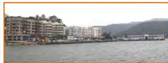
梅窩渡輪碼頭及 鄰近住宅發展 Mui Wo Ferry Pier & nearby residential developments
