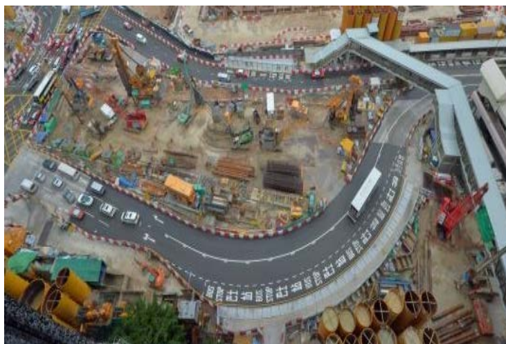
Carriageways of the section of Convention Avenue between Expo Drive, Expo Drive East and Fleming Road were shifted northward
