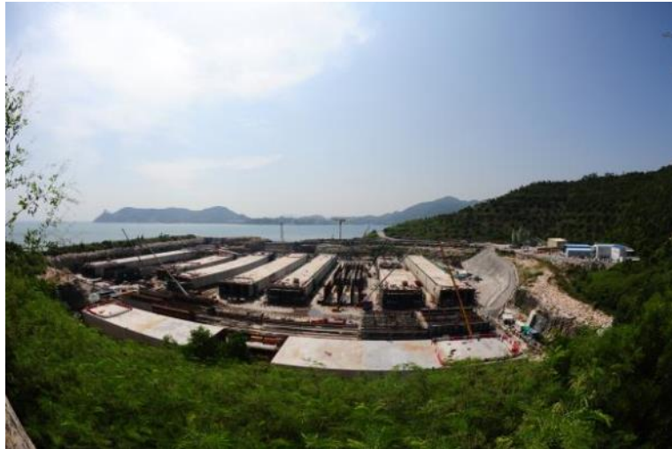
Casting yard of IMT pre-cast units
