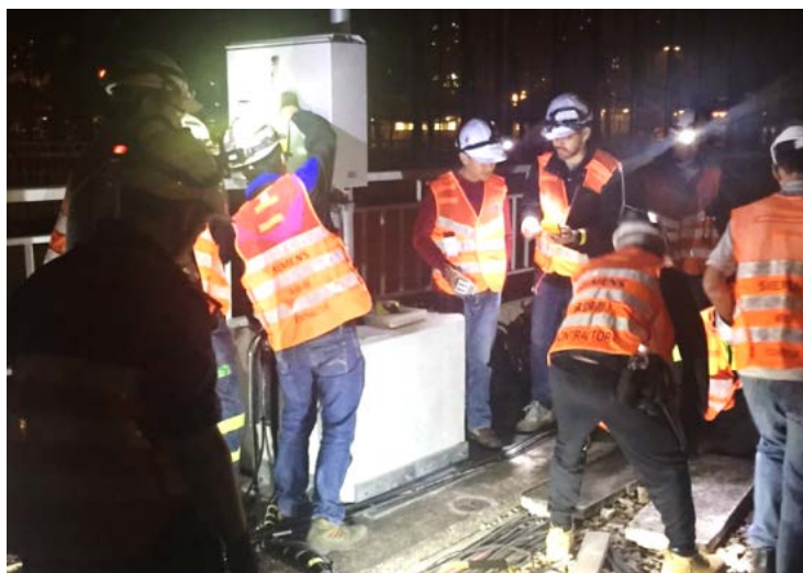
Signalling upgrade along EAL
