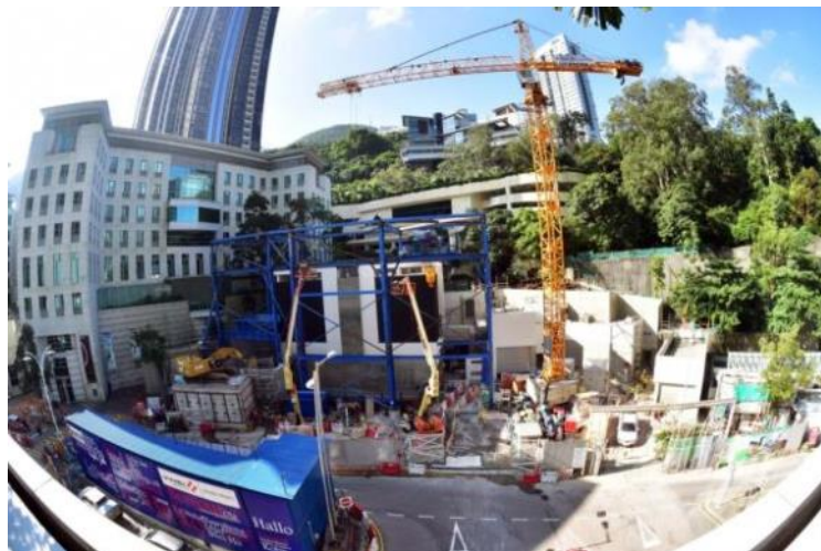
SCL overrun tunnel construction site at Hong Kong Park
