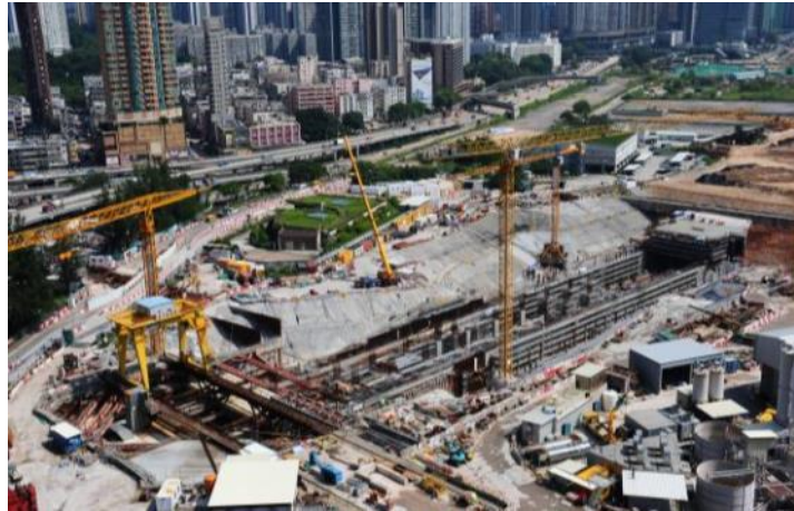
Structural works for To Kwa Wan Station
