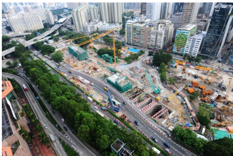
Structural works Expansion works for Diamond Hill Station
