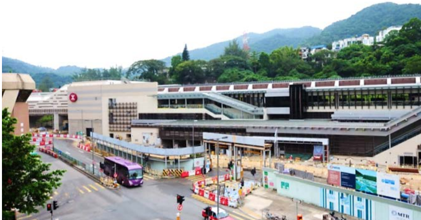
Hin Keng Station and part of the viaduct
