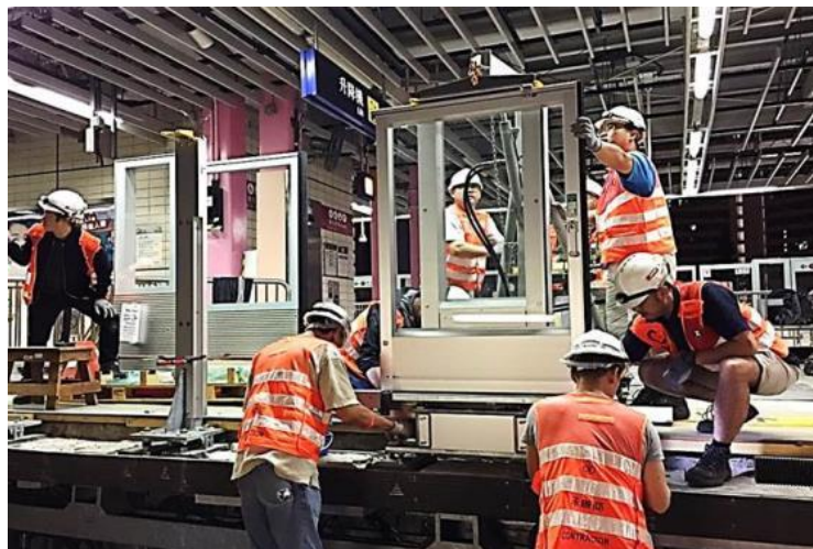
Retrofitting works of APGs
