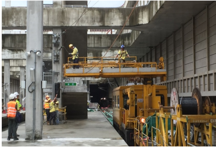
Overhead line at ERS is ready for the first XRL train's dynamic testing along the pilot test section
