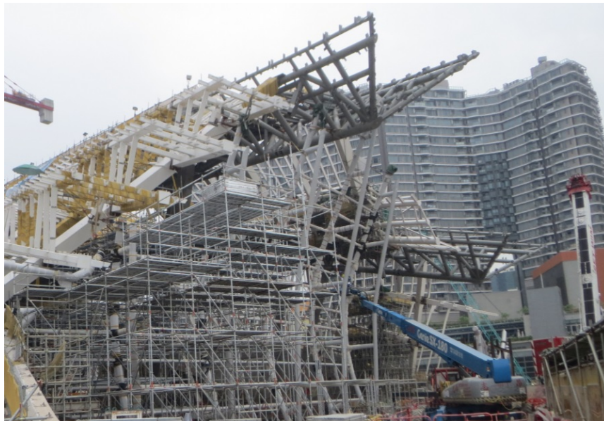
The facade at the southern side of the Station Entrance Building
