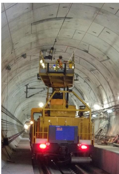
OHL wire stringing in tunnel
