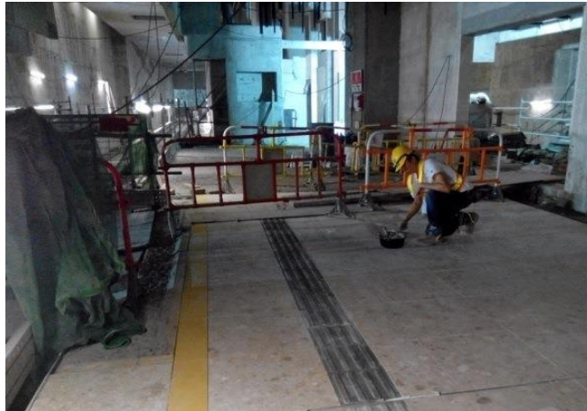
Floor finishing at WKT platform level
