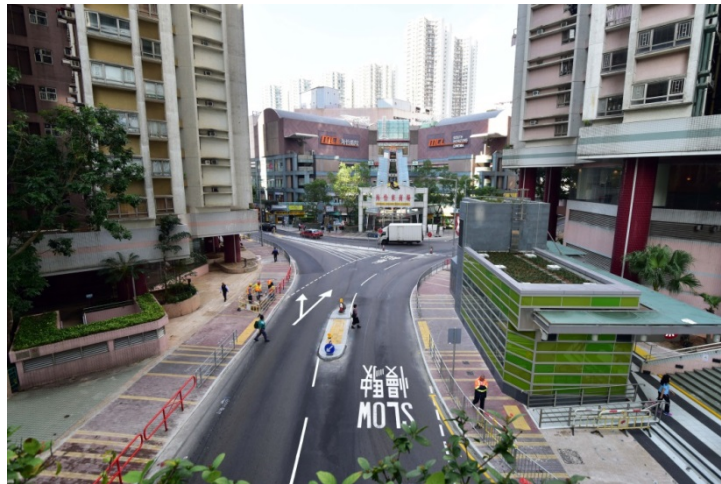
Remaining footpath reinstatement works in progress in South Horizons
